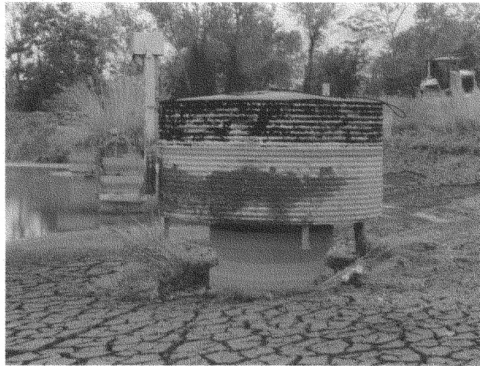
Photo B-4: Old Spillway Weir (to be abandoned)
