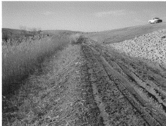
Photo C-4: As Found Conditions of Paradise Gypsum Stack South Slope
