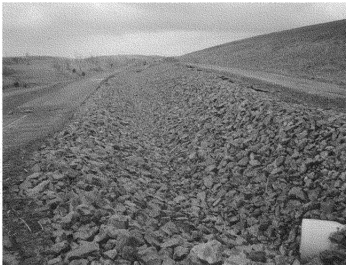
Photo C-5: May 2009 – Renovations Completed to Control Seepage and Surface Runoff
