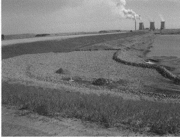
Photo C-3: April 2009 – West End of Rock Butress Completed
