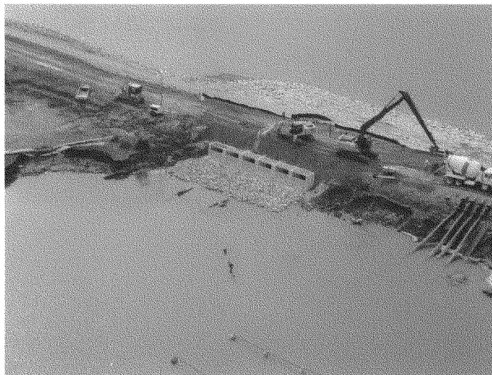
Photo B-2: New Spillway and Siphon Systems (viewed from upstream)
