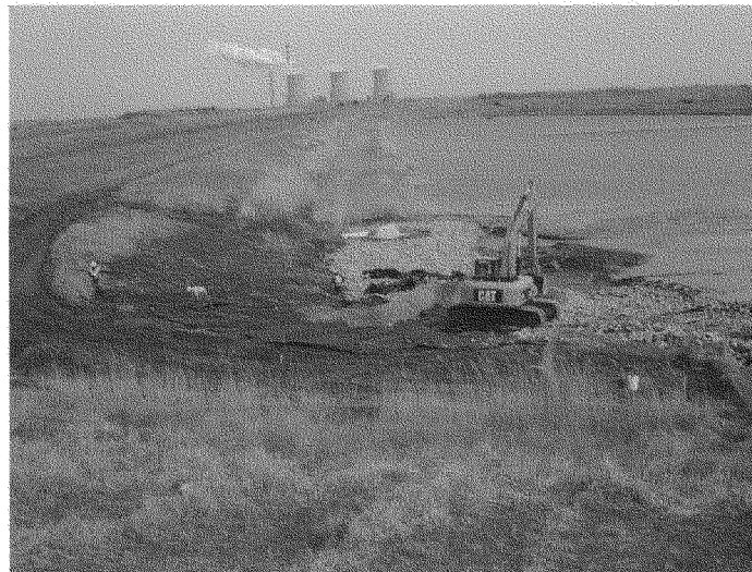
Photo C-2: March 2009 – Beginning Construction of Rock Buttress to Stabilize Slope
