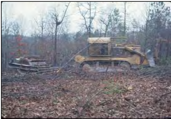
Figure 1. Drum chopper pulled by a bulldozer.
