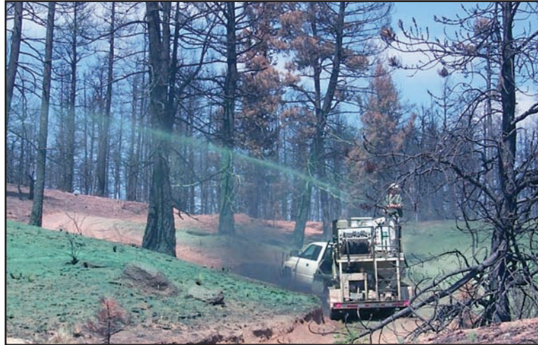
Figure 22. Trailer-mounted sprayer used to apply hydromulch from the road as a post-fire hillslope treatment on the 2002 Hayman Fire in Colorado.
