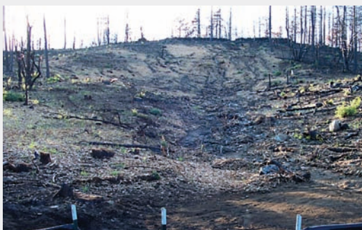
SB3-fig. 1. Wood chips used for post-fire hillslope treatment. Note that wood chips that were entrained in the overland flow are piled at the outlet of the swale.
