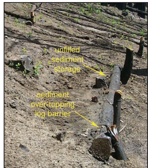
Figure 14. A partially filled LEB with unused sediment storage capacity indicated.
