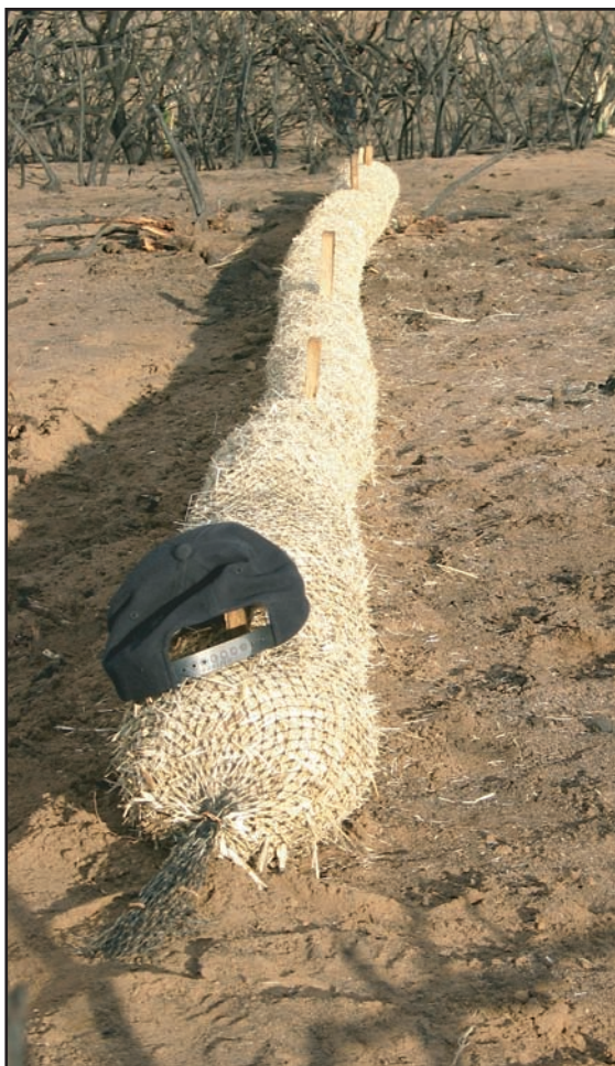
Figure 9. A recently installed straw wattle erosion barrier.
