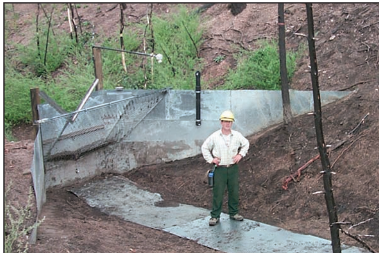
Figure 7. Cleaned-out sediment basin at the outlet of a catchment study site on the 2002 Hayman Fire in Colorado.
