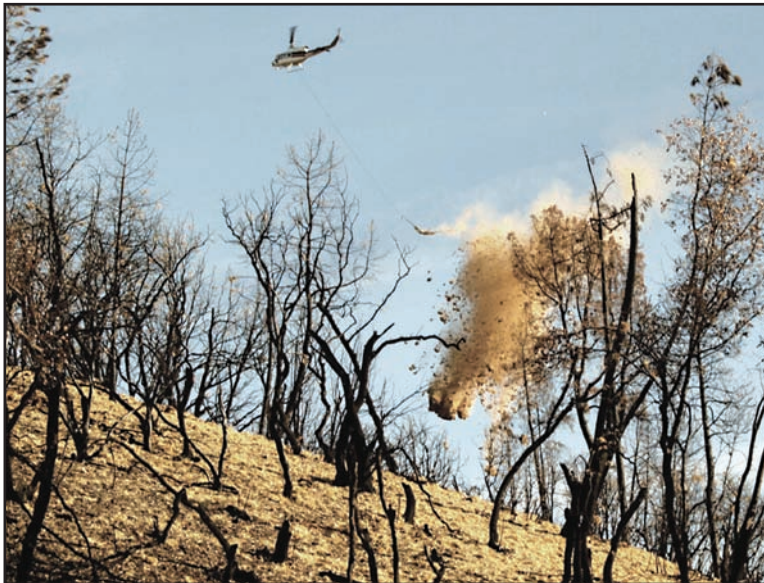
Figure 20. Aerial application of post-fire straw mulch treatment using a cargo net suspended below a helicopter; the cargo net is released over the target area (photo from Napper 2006: 25).
