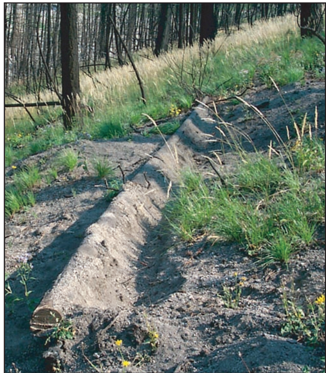
Figure 8. A contour-felled log erosion barrier with soil end berms to increase sediment storage capacity.
