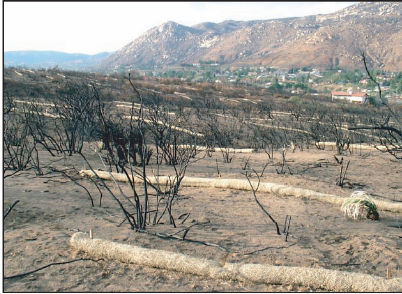
Figure 11. Straw wattles installed in a staggered layout on a burned hillslope.
