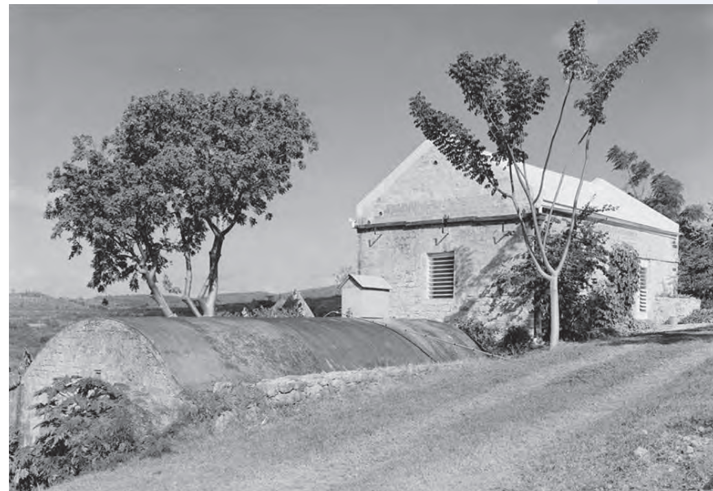
partially underground cistern
