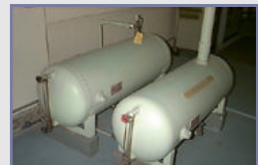
Fig. 1: Investigate storage tanks as part of the plumbing system review
