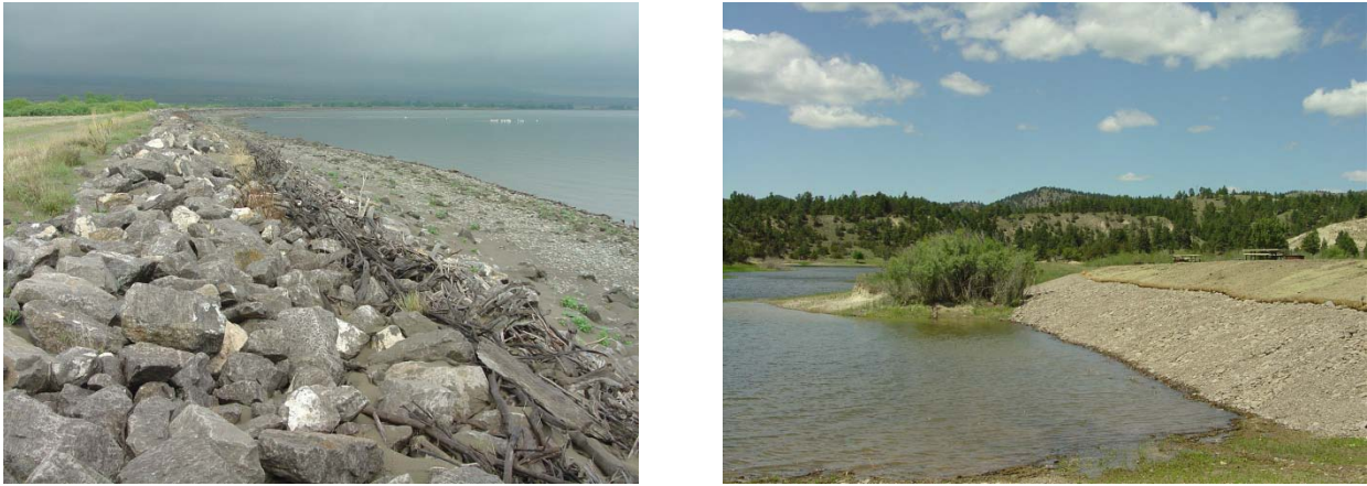
Figure 6. Examples of riprap at Canyon Ferry Reservoir.
