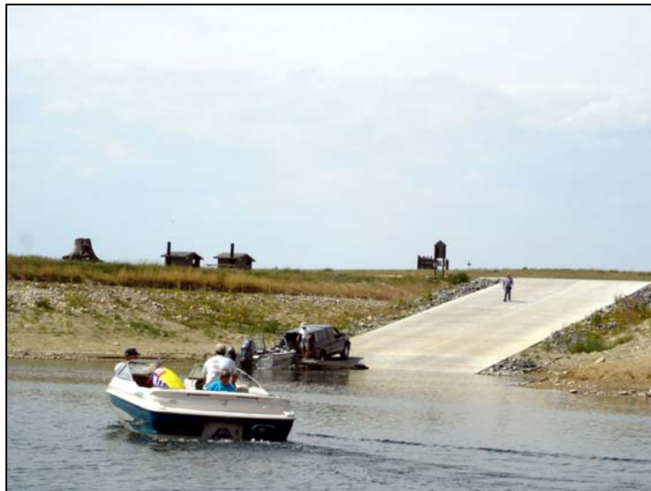
Figure 10. Goose Bay Boat Launch Ramp & Toilets
