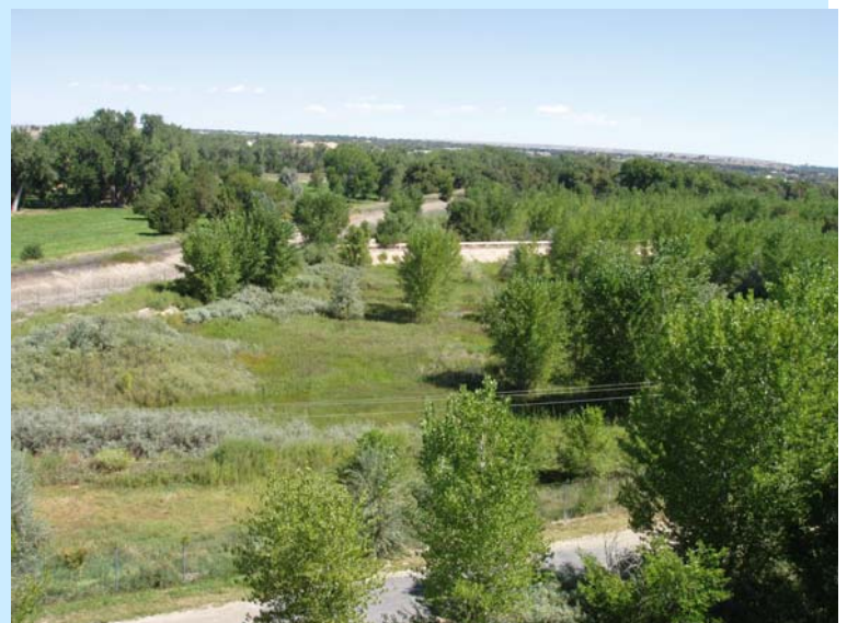
Site for water treatment facilities near existing Whitlock Water Treatment Plant.
