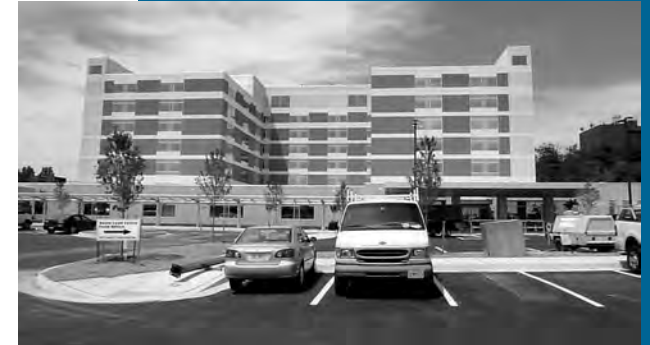
Franklin Square Hospital, a CCP Partnership site, is nearly completed.
