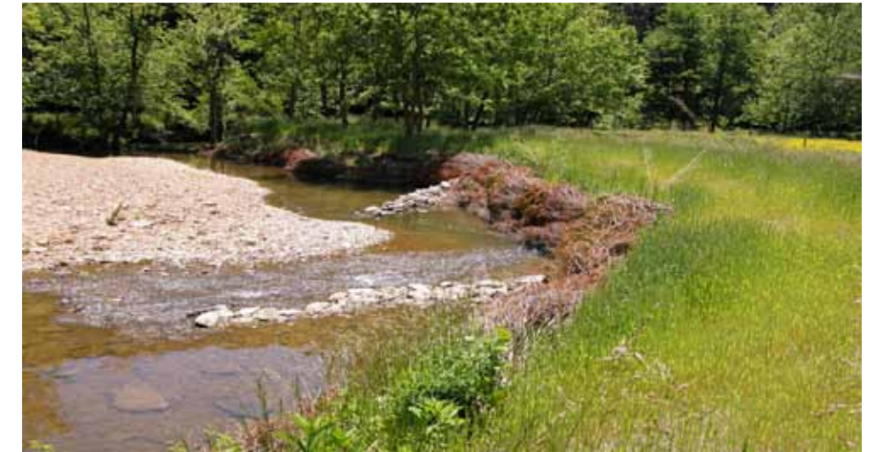
A protected and restored streambank with in-stream structures, Kentucky
