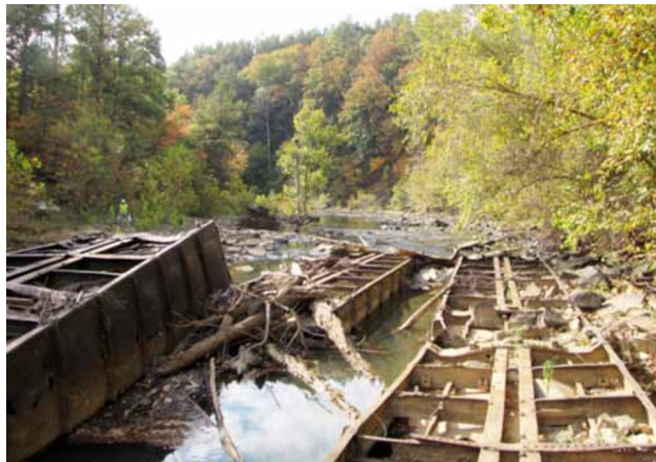
Abandoned parts from old rail cars, formerly the base for a construction road crossing Shades Creek, blocking and redirecting stream flow and creating a fish passage obstacle, USFWS.
