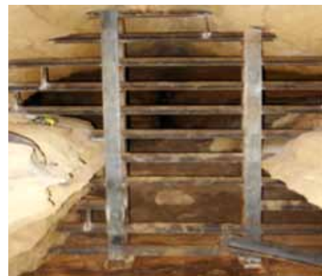
A completed cave gate structure
