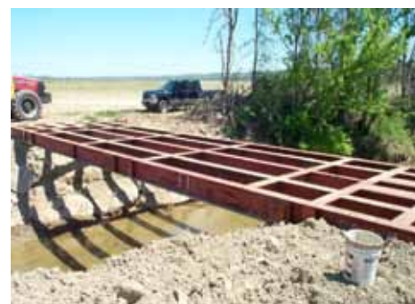
Stream crossing following culvert removal, USFWS.
