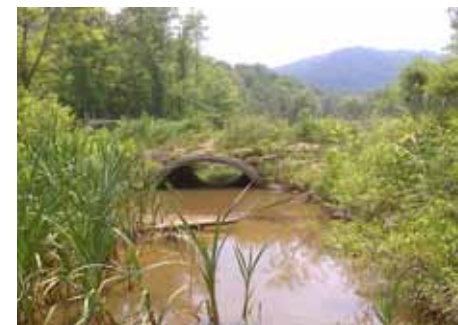
Top: fish passage barrier and degraded stream habitat negatively affecting (T) blackside dace; below: after fish barrier has been removed, 2300 feet of stream restored and replaced with a fish friendly passage, USFWS.
