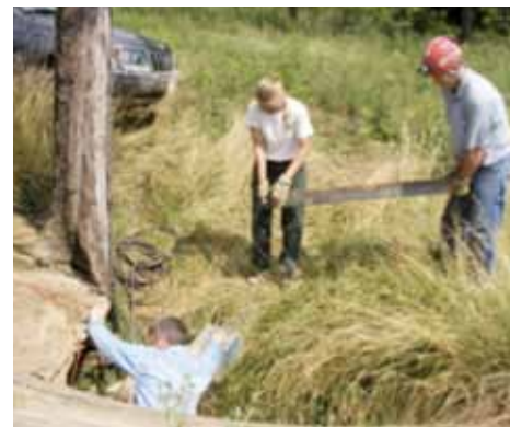
Installing a cave gate
