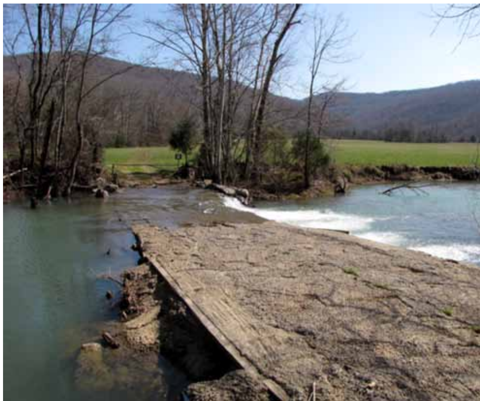
Low water ford on Hurricane Creek, a tributary to the Paint Rock River in the Tennessee River Basin. This ford was targeted for removal through an assessment of all road crossings in the watershed with the potential to act as a fish passage barrier; USFWS.
