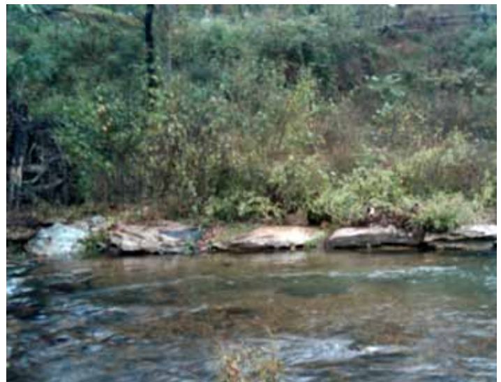
After: stream following removal of low dam on Tennessee stream
