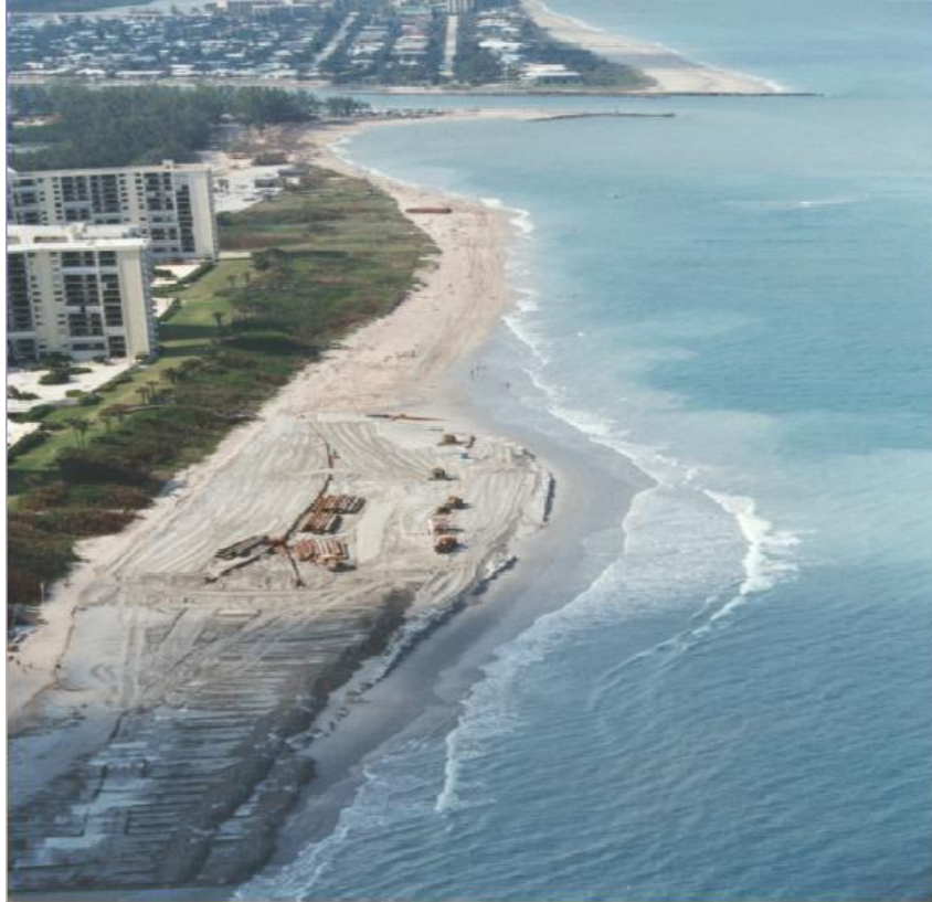
Figure 3: Example of a typical beach renourishment project, Palm Beach County, Florida. (Photo provided by Palm Beach County Department of Environmental Resources Management).
