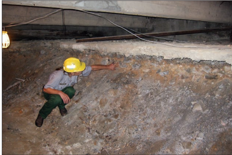
Basement investigations at the Ozark Bathhouse.
