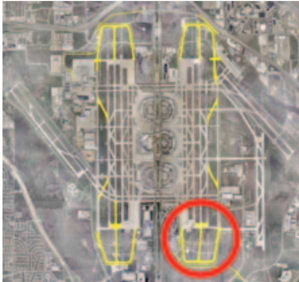
Perimeter taxiway in the South East quadrant opened in December 2008 at Dallas/Fort Worth International Airport
