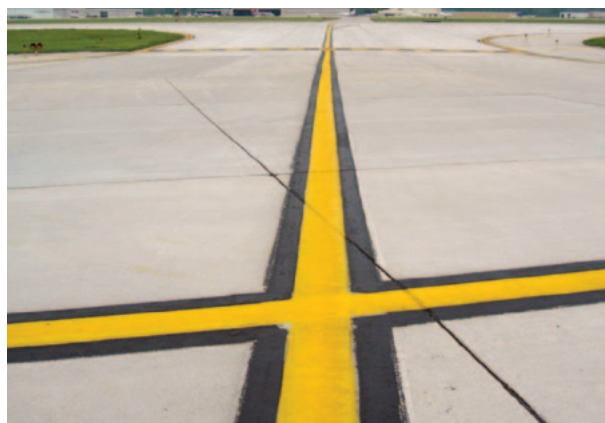
Previous Taxiway Centerline Markings
