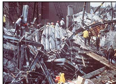
Figure 4. Rubble after the L,Ambiance Plaza collapse in 1987. Photo credit National Institute of Standards and Technology
