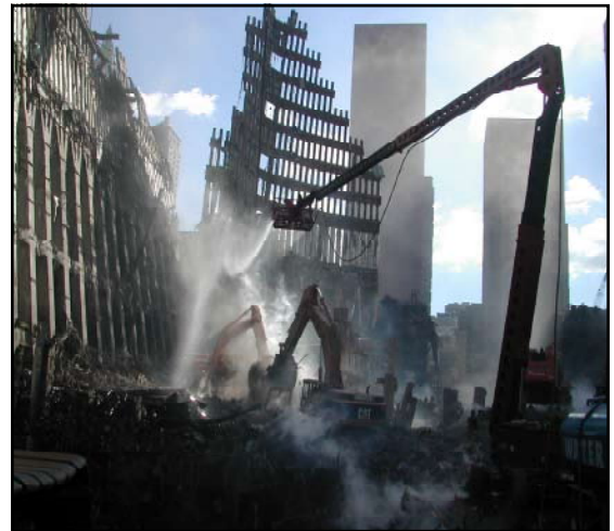
Figure 9. Operating Engineers removing debris at WTC.
