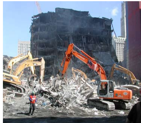
Figure 3. Operating Engineers at Ground Zero.
