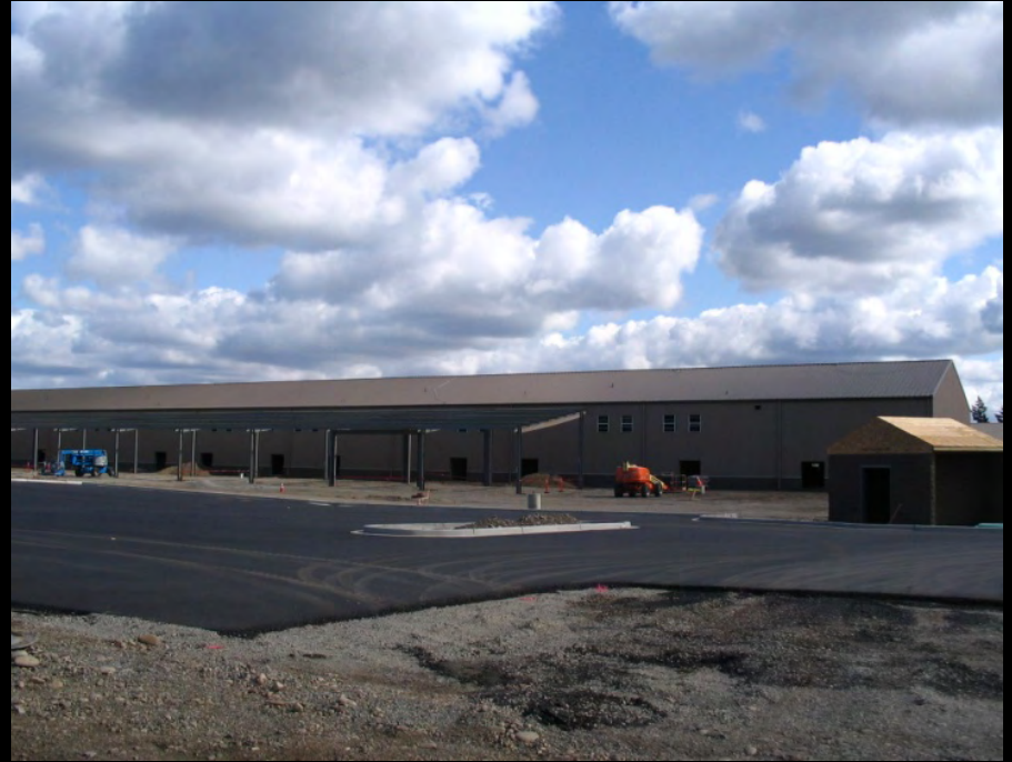
Company Operations Facility, Fort Lewis, FY07
