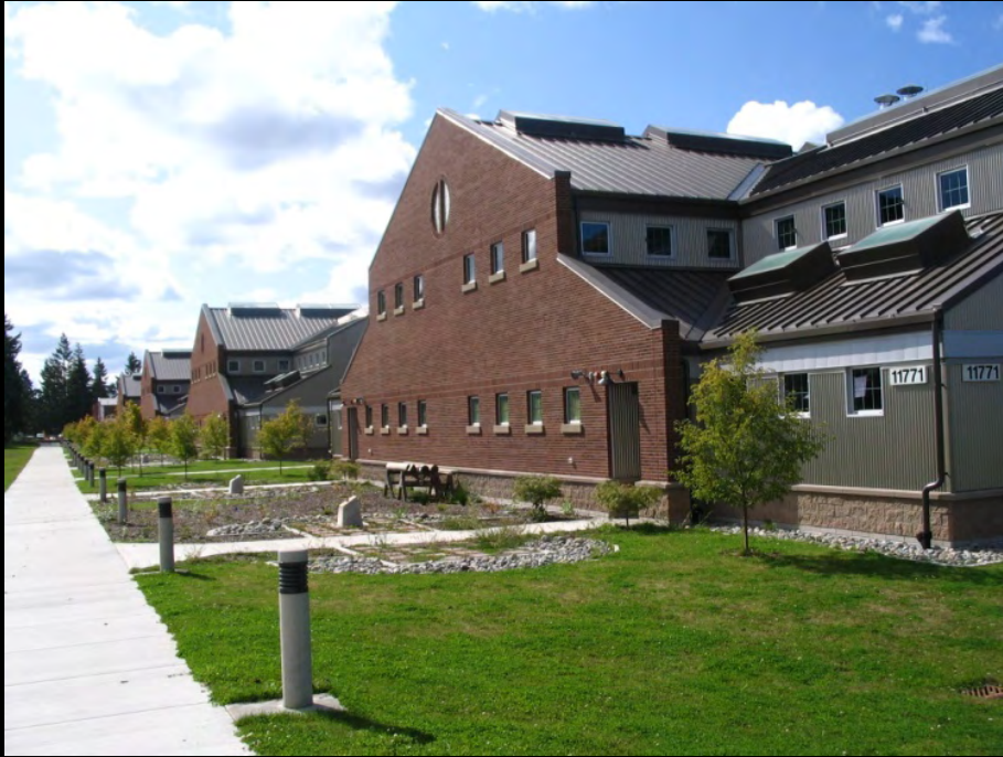
Company Operations Facility, Fort Lewis, FY05
