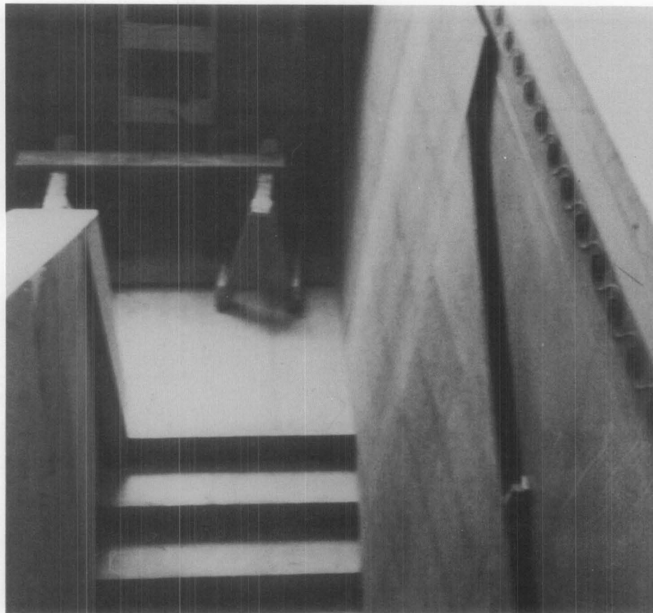
Figure 6. The balustrade on the left side of the photograph has been entirely encased in plywood to protect it from damage. Note that the kick-out at the end is due to the protrusion of the newel post. Photo: Charles Fisher.
