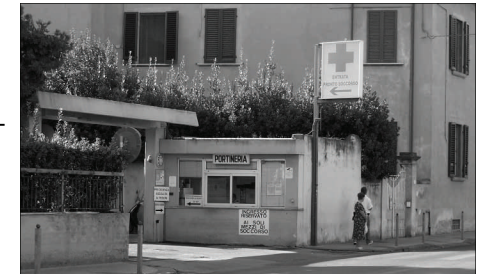
Emergency entrance on Via Bonanno Pisano
