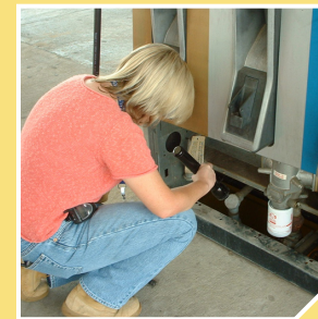
Inspecting under the dispenser
