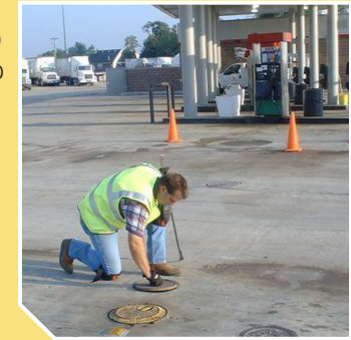
Inspecting a spill bucket
