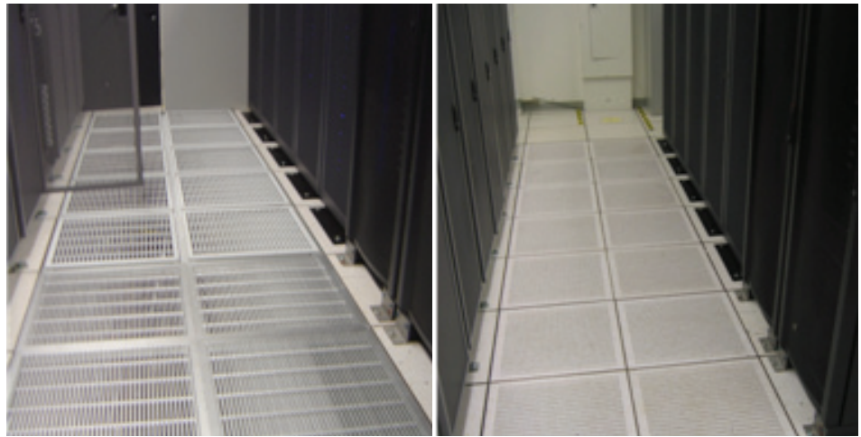
Figure 8: Floor tiles; before and after retrofit
