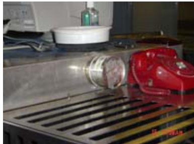
Photos 26-29: Examples of blocked emergency buttons
