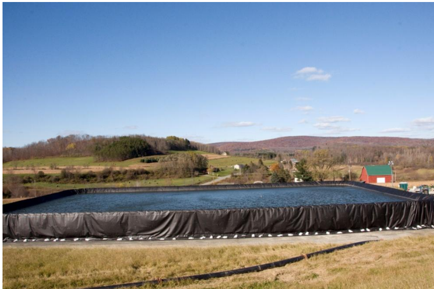
A temporary freshwater impoundment to be used for fracking, or hydraulic fracturing.
