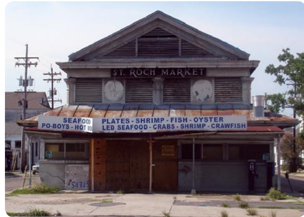
The St. Roch Market, a historic institution, has been closed since the storm, but community leaders would like to bring a farmers’ market back to the building to provide fruits and vegetables for the neighborhood.
