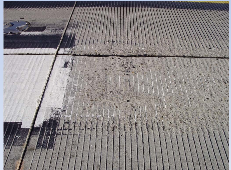
Visible pavement scars caused by grinding of paint markings.
