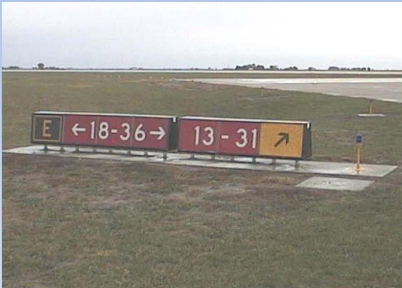
Direction sign arrow on a holding position sign
