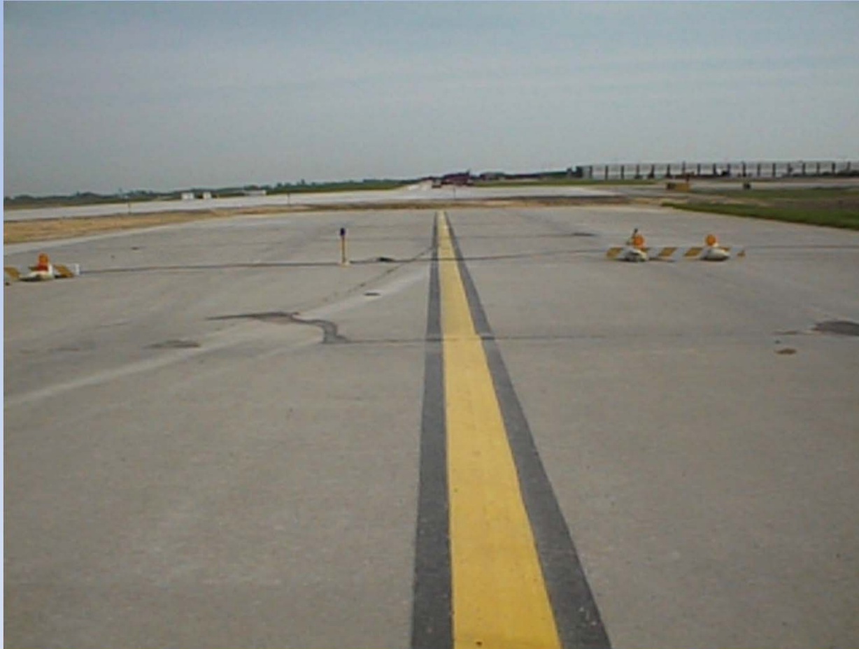
Taxiway centerline leading into a dead end construction zone.
