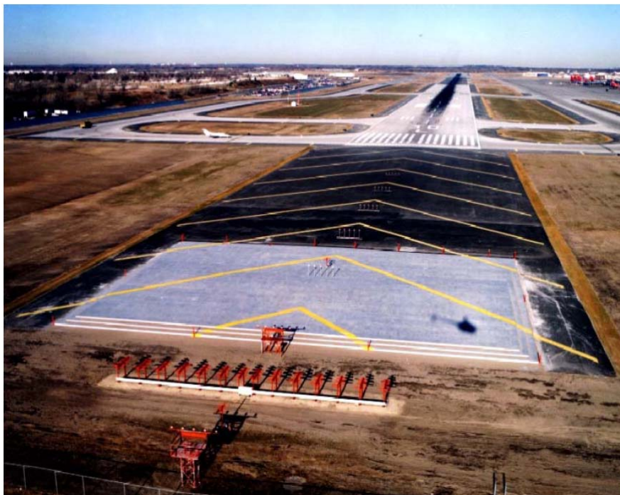
FIG AD 1.1-54 Engineered Materials Arresting System (EMAS)
