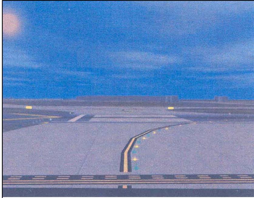
FIG AD 1.1-12 Taxiway Lead-On Light Configuration
