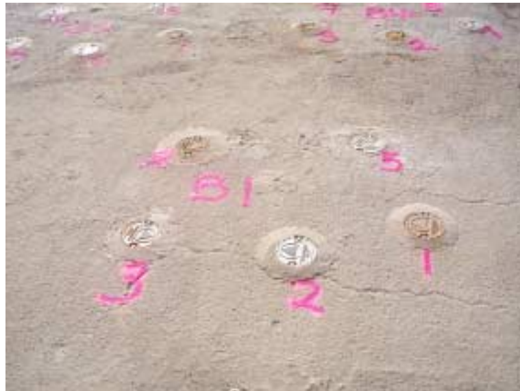
Image 12. Completed wells within Cell B.
