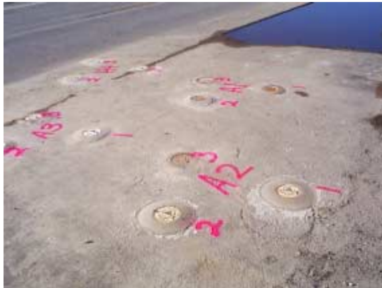
Image 11. Completed wells within Cell A.
