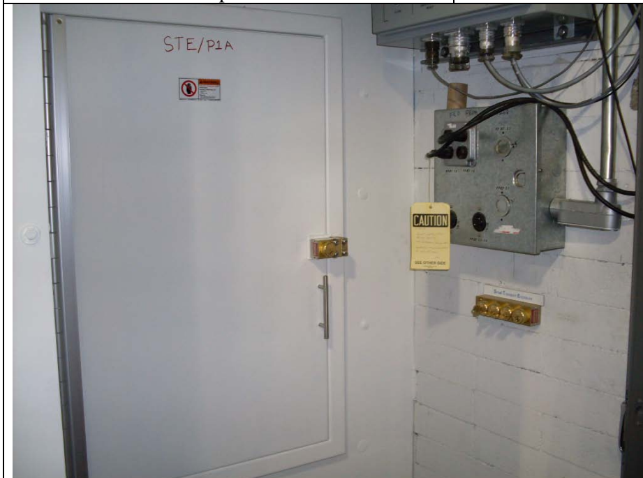
Figure 4: STE Upstream Access panel and STE Transfer Key Bank
