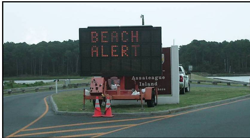
Figure 33. VMS Location During Tropical Storm Danny.
