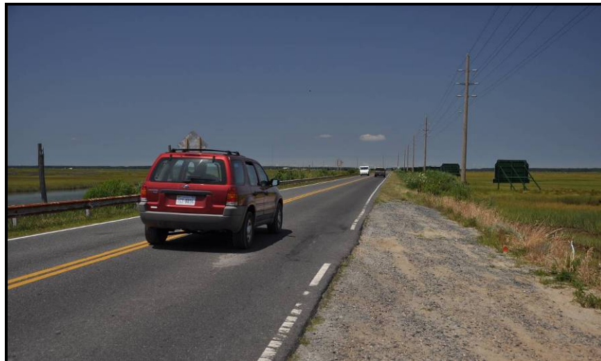
Figure 9. Route 175 Causeway (looking west toward the mainland).
