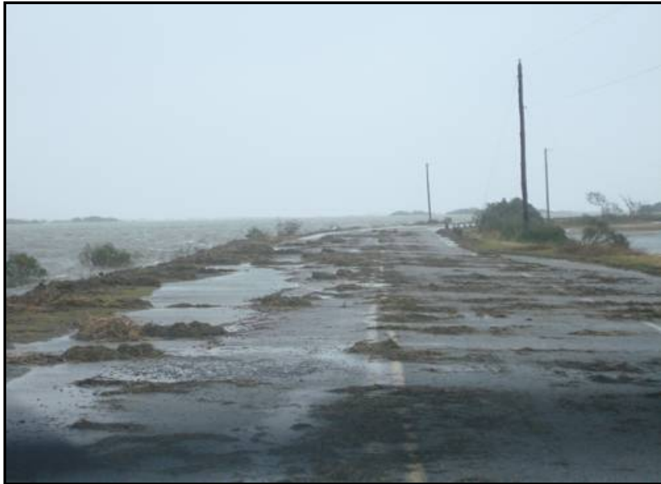
Figure 2. Beach Road Post-Storm, November 2009.
