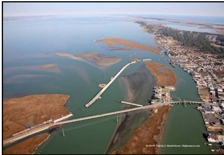
Figure 36. Route 175 Bridge Construction, Aerial Photo, January 2009.
