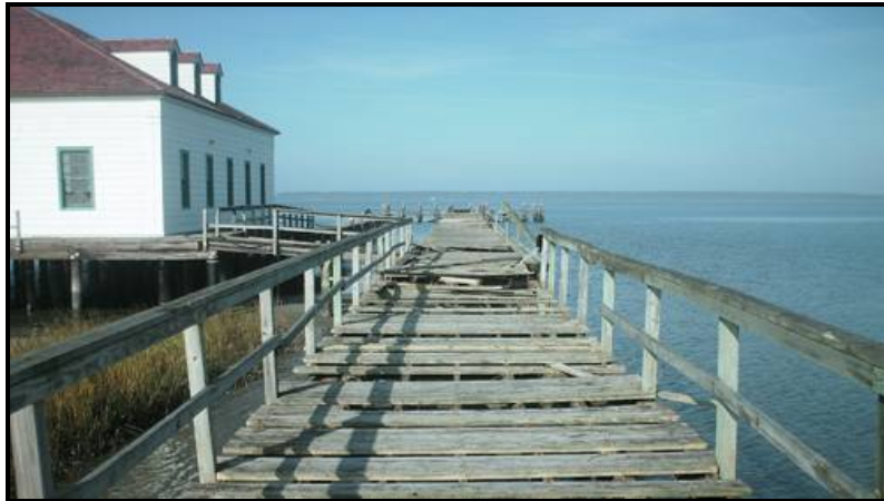
Figure 31. Former U.S. Coast Guard Station (Toms Cove).
