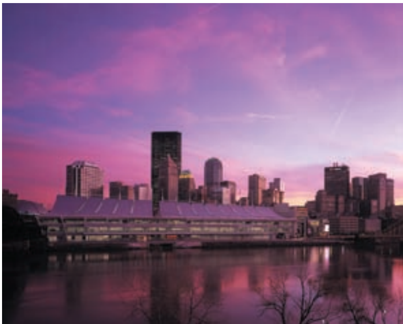
Pittsburgh's David L. Lawrence Convention Center opened in September 2003 as the world's first certified "green" convention center. Encompassing nearly 1.5 million square feet on a former "brownfield" site adjacent to public transportation routes, its daylighting design provides natural light for 75 percent of the convention center's exhibition space, saving 9.5 million kWh of electricity a year. The building uses about 35 percent less energy than a conventionally designed building of comparable size. 33
