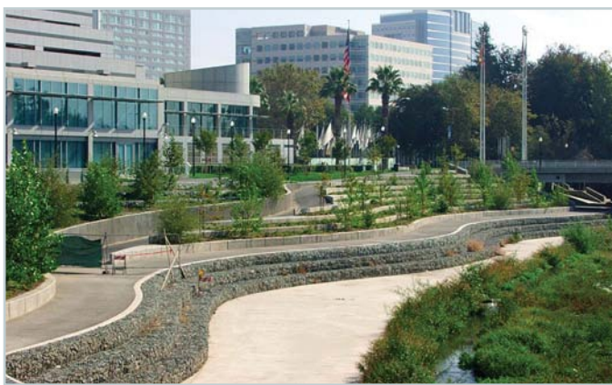
Figure 1: Guadalupe River Park in San Jose, California, features green infrastructure systems alongside dense downtown redevelopment. Photo courtesy of Michael Patrick via Flickr: http://www.flickr.com/photos/michaelpatrick/2408259482/ .
