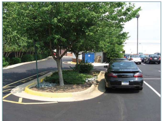
Figure 1: Bioretention areas, like the one in this parking lot, are commonly used in Stafford County to meet local stormwater requirements.
