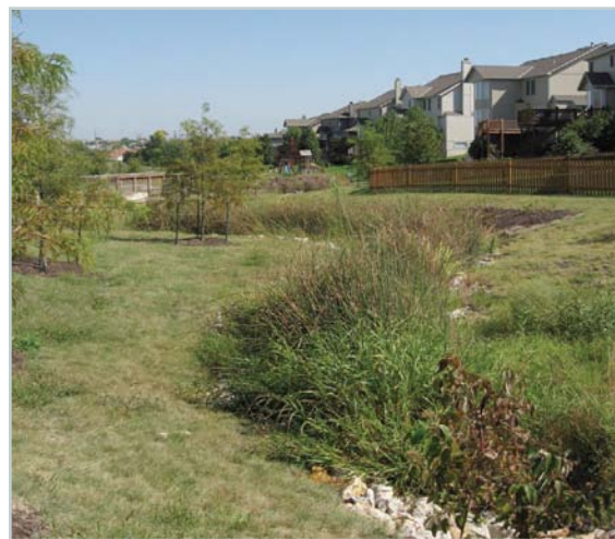
Figure 1: A constructed 1 st order intermittent stream in a neighborhood development slows and infiltrates stormwater runoff, while adding aesthetic value for residents. Plant selection and landscape transition plantings were carefully considered for acceptance.
