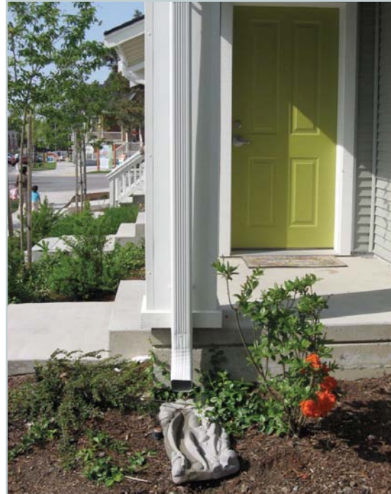
Figure 13: A disconnected downspout in Seattle, Washington.
