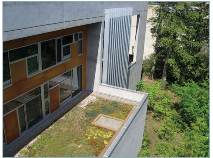
Figure 1: A green roof at Evergreen College was built to offset the addition of new impervious surfaces from new parking spaces.
