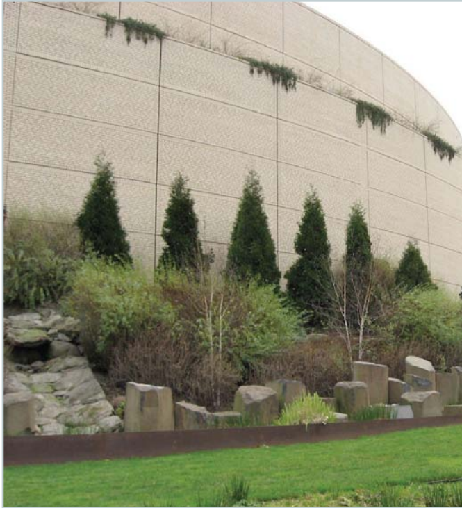
Figure 12: Oregon Convention Center saves $15,600 per year on its stormwater bill by managing roof runoff in these rain gardens.
