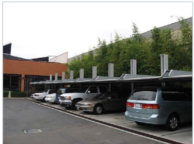
Figure 2: Multi-level or stacked parking behind a business further reduces imperviousness and complies with Emeryville’s “Stormwater Guidelines for Green, Dense Redevelopment.”
