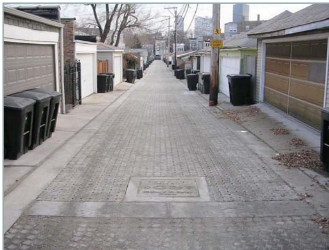
Figure 1: Chicago's Green Alley Program retrofits existing alleyways to include permeable pavers like these to infiltrate stormwater runoff. Photo courtesy of David Leopold.
