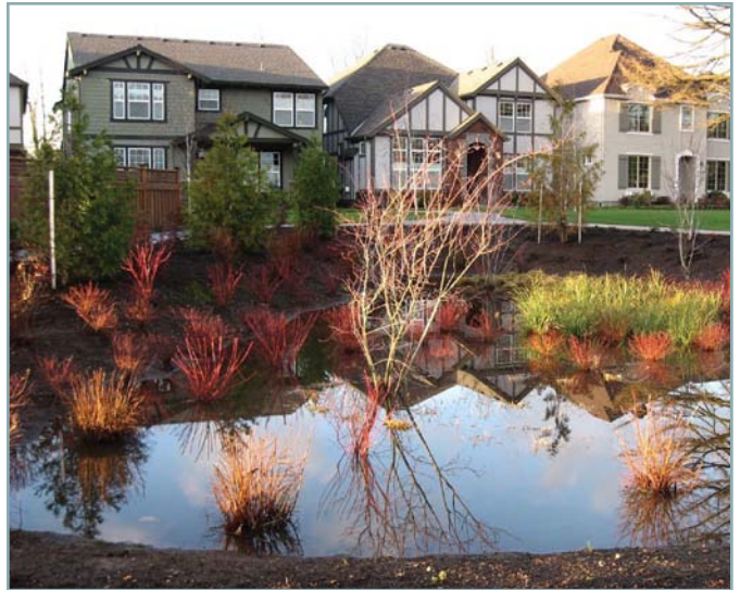
Figure 2: Decentralized stormwater management features, such as this bioretention area in the Villebois project, collect runoff from rooftops, sidewalks, and yards for infiltration into the ground below.
