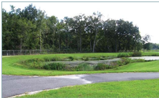
Figure 2: Depot Pond is a former brownfield site that was cleared of contaminated soil and converted into a functional wetland for managing runoff from nearby downtown.
