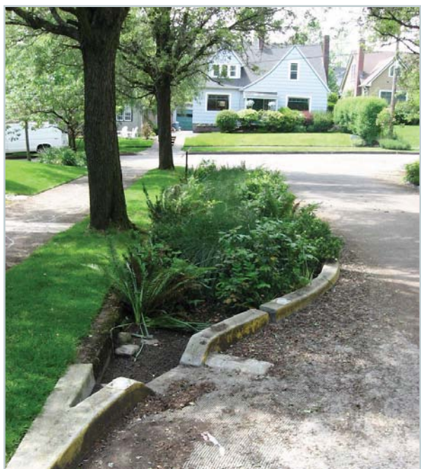
Figure 2: Portland’s first Green Streets project at NE 35th and Siskiyou features curb cuts, bump outs and swales.
