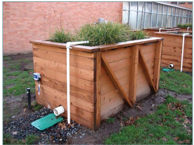
Figure 1: The City of Wilsonville worked with developers to monitor the performance of new green infrastructure techniques, like this planter box, before establishing development standards for on-site management.
