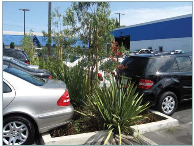
Figure 1: This commercial site includes parking lot swales to bioinfiltrate impervious surface runoff.
