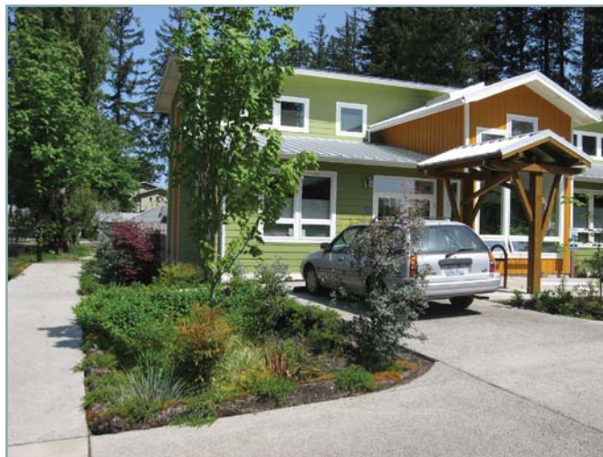
Figure 2: A medical center in Olympia, Washington, manages runoff from the roof and other impervious areas through small swales and permeable sidewalks.
