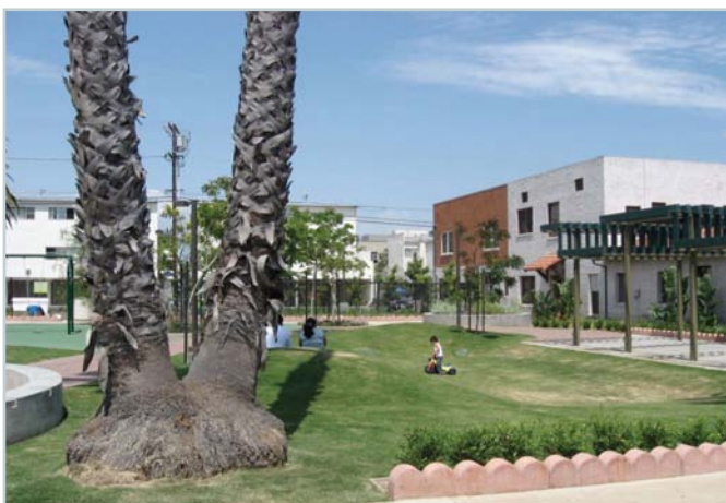
Figure 3: Euclid Park in Santa Monica, California, includes a depressed area with storage underneath, doubling as a public amenity and stormwater structure.
