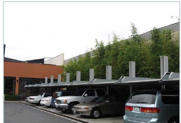
Figure 5: All developers in Emeryville, California, must comply with the City's "Stormwater Guidelines for Green, Dense Redevelopment," which requires green infrastructure, such as this stacked parking lot, throughout a project's planning and operation.
