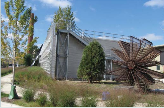
Figure 2: This Chicago building features a green roof, permeable pavers and bioswales, which meet Chicago's stormwater management requirements.
