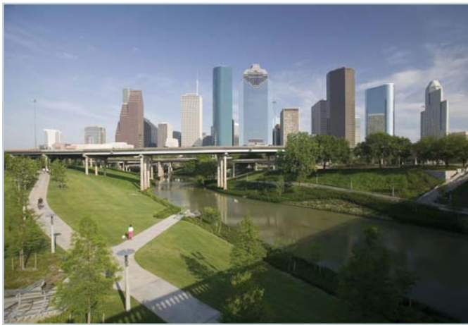
Figure 4: The Buffalo Bayou Promenade in Houston, Texas, retrofitted a formerly impervious area and restored this major drainage way as green infrastructure. The Bayou now has improved floodwater conveyance, in addition to providing other community and environmental benefits. Photo courtesy of Tom Fox, http://www.asla.org/2009awards/104.html .
