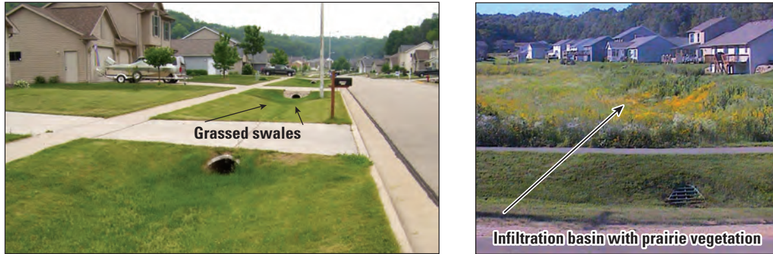
Figure 3. Example of stormwater-runoff controls using low-impact-development practices.
