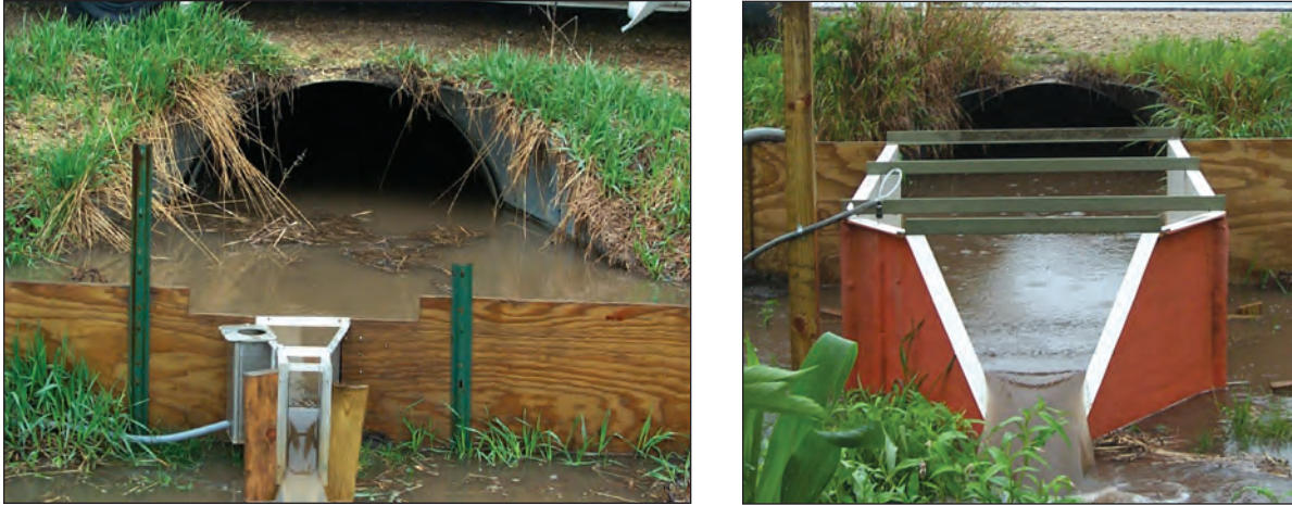
Figure 4. Parshall flume (left) used to measure discharge at the low-impact-development (LID) basin outlet. The Parshall flume was later replaced by an H-flume (right) to accommodate larger discharge events.
