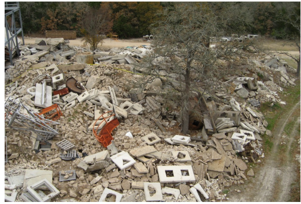
Figure 1: Concrete rubble pile training scenario which simulates a fully collapsed concrete structure.
