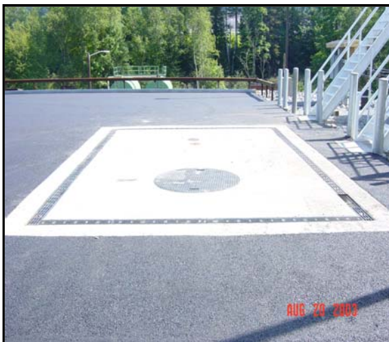
Figure 6. Flat pad containment system (Photograph by C&S Engineers, Inc., courtesy of New York State Department of Correctional Services.)
