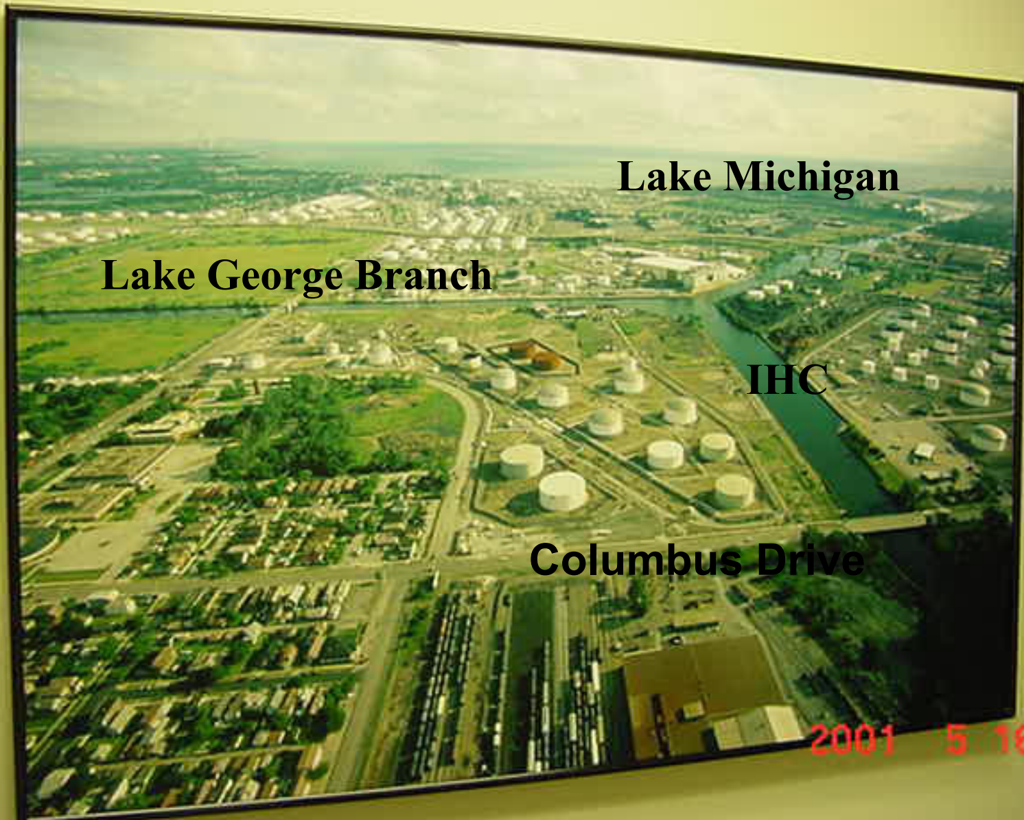
Overview of Canal System
