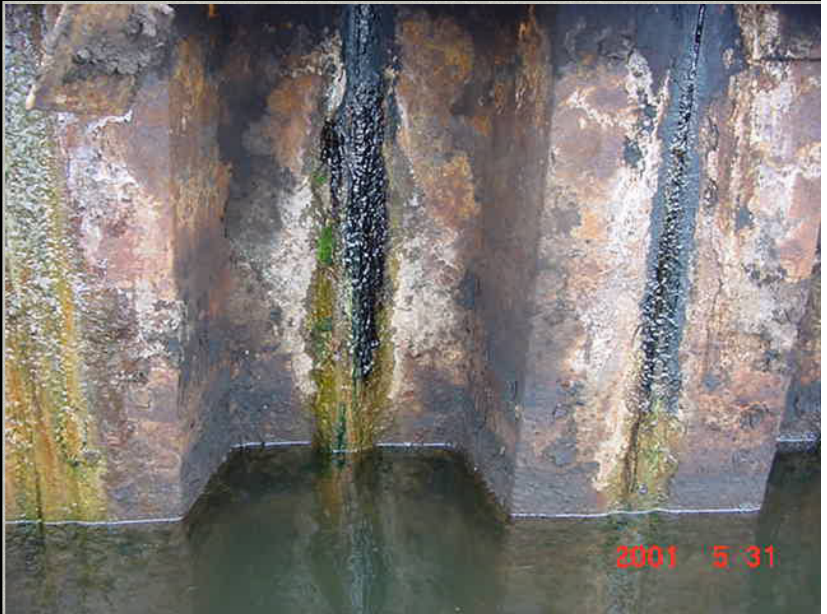
More sheet piling
