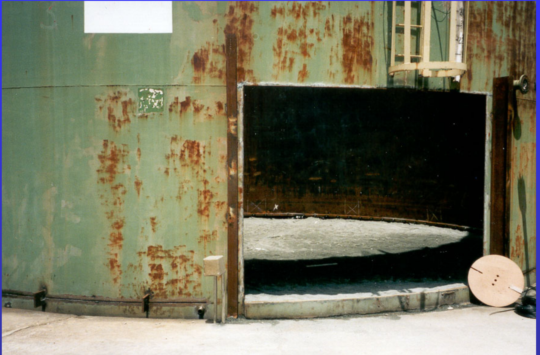
New Floor Installation on Existing AST
