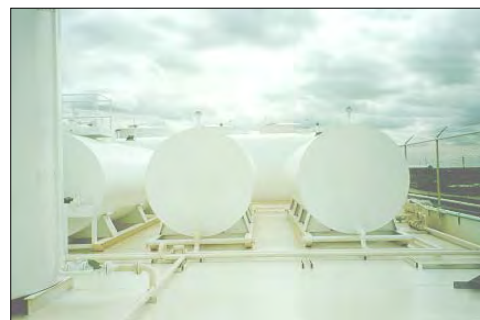
Figure 7-3. Shop-built containers elevated on saddles.
