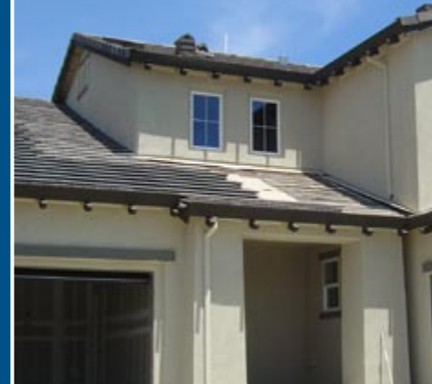
Low Riders: Builders and homeowners prefer collectors and arrays that hug the roof line.
