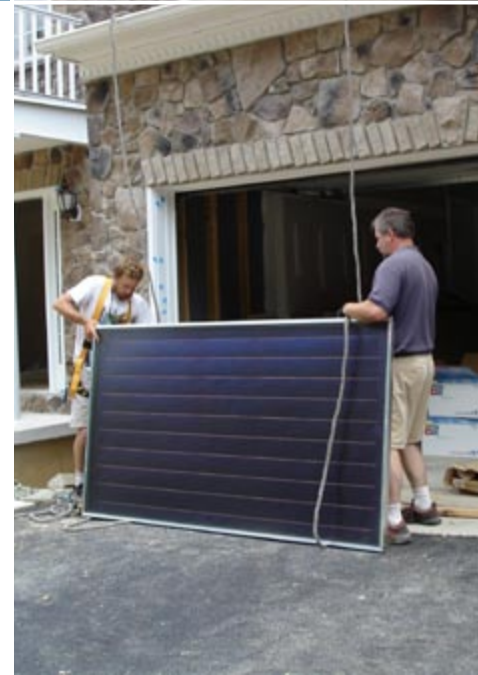
Installers prepare to lift a solar panel onto the roof.
