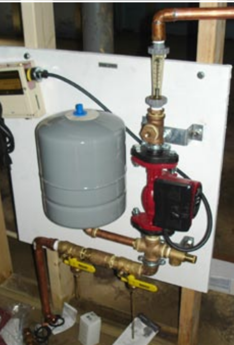
(left, middle, right) Field-mounted gauges, pumps, and valves and an example of a prepackaged unit.
