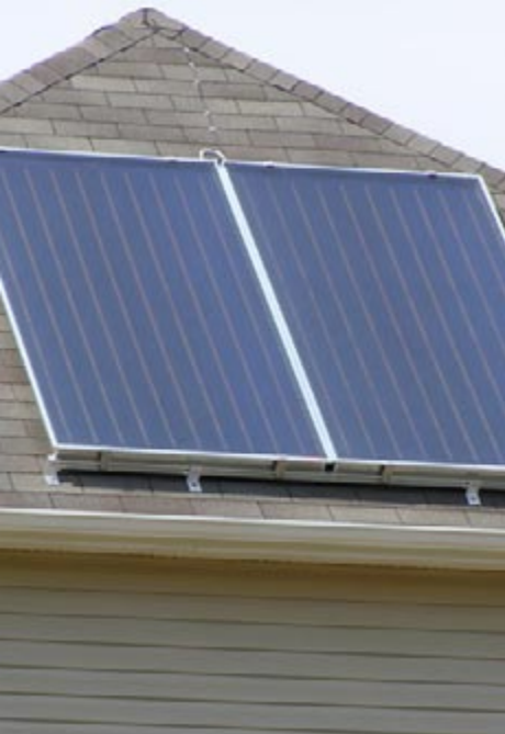
(left) Glazed flat plate collector.
