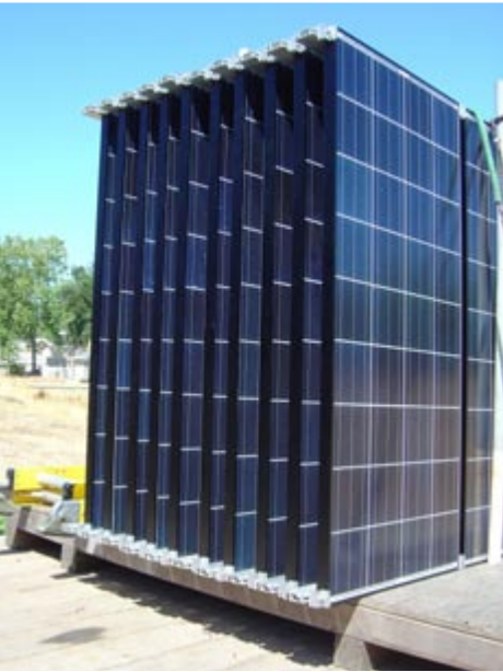
(left) Photovoltaic installers have attached mounting rails to the PV modules in the shop. This saves time on the roof and provides for easier shipping.
