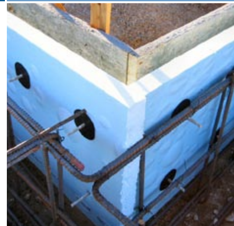
Clarum is building four zero energy research homes at Borrego Springs, California. Polystyrene slab edge insulation helps to carefully control heat gains and losses. Photos courtesy of Clarum Homes.
