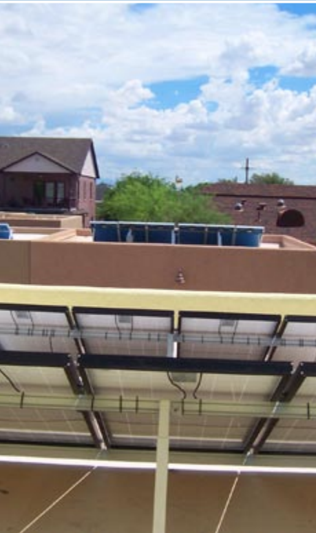
All homes come standard with a 1.5-kW photovoltaic system and solar hot water collector. (left) Photo courtesy of NAHBRC. (right) Photo courtesy of JWM.
