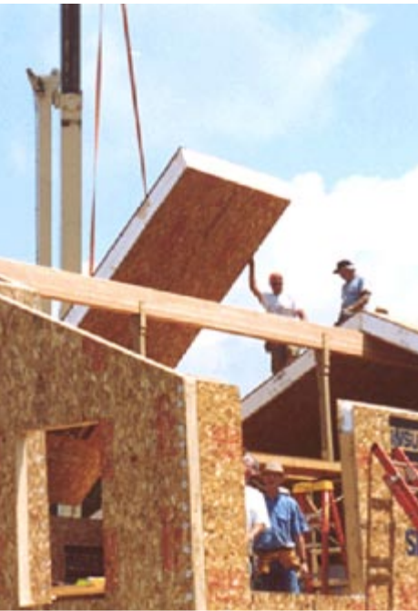
(left) All five houses use structural insulated panels (SIPs) for super-efficient wall and roof construction.
