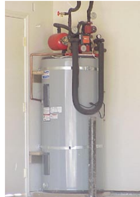
(left) Rough-in plumbing for a solar thermal system. Photo courtesy of Heliodyne.
