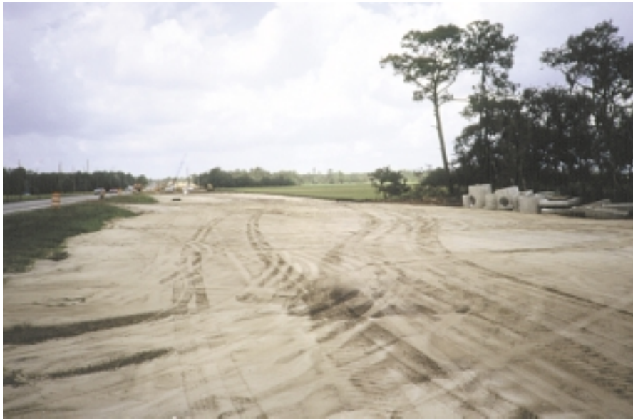
Figure 17. Two examples of development in coastal areas. A) A highway project resulted in placement of fill in estuarine emergent wetlands in coastal Georgia, 1995, and B) an estuarine emergent marsh was filled for a new development in coastal Texas. (B, U.S. Fish and Wildlife Service: J. Dick)
