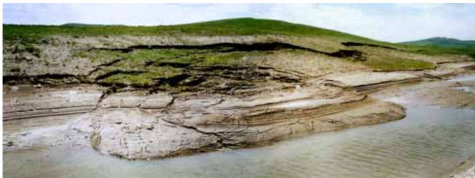
Figure 1: One of 16 documented slides on the St. Mary Canal.
