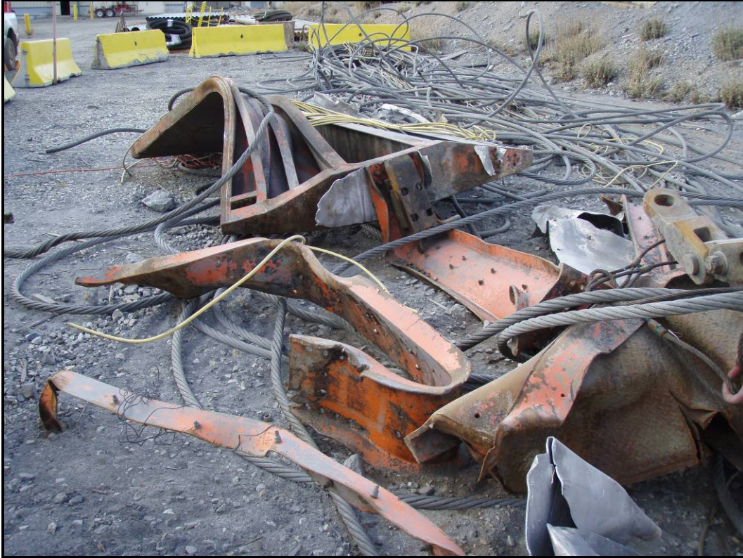
Photo 5 – Damage to hoist platform and other hoist components.
