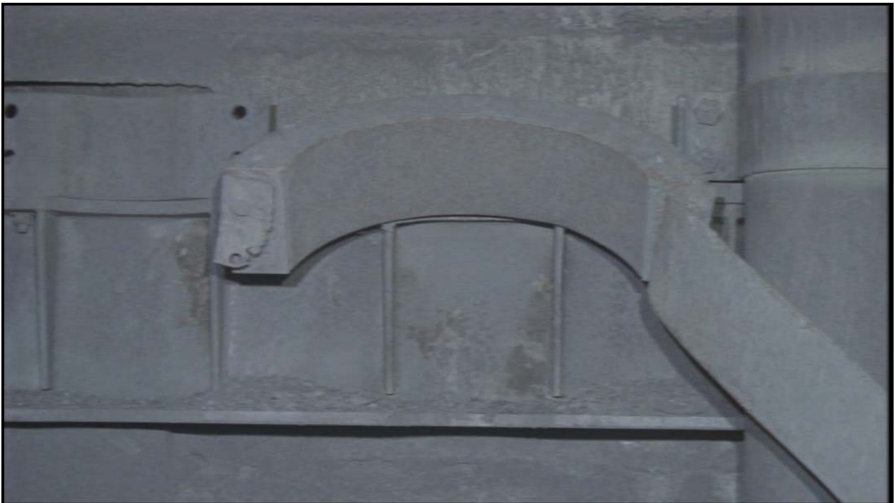
Photo 24 – Video Time 1:23:20 – Bearing clamp sheared at a location 472 feet from the collar.
