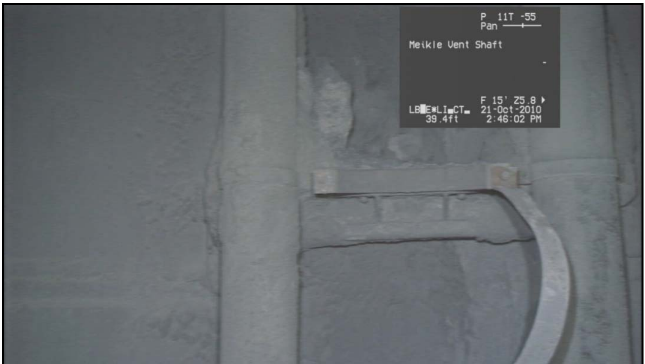
Photo 18 – Video Time 6:17 - Original bracket with one clamp bolt sheared.
