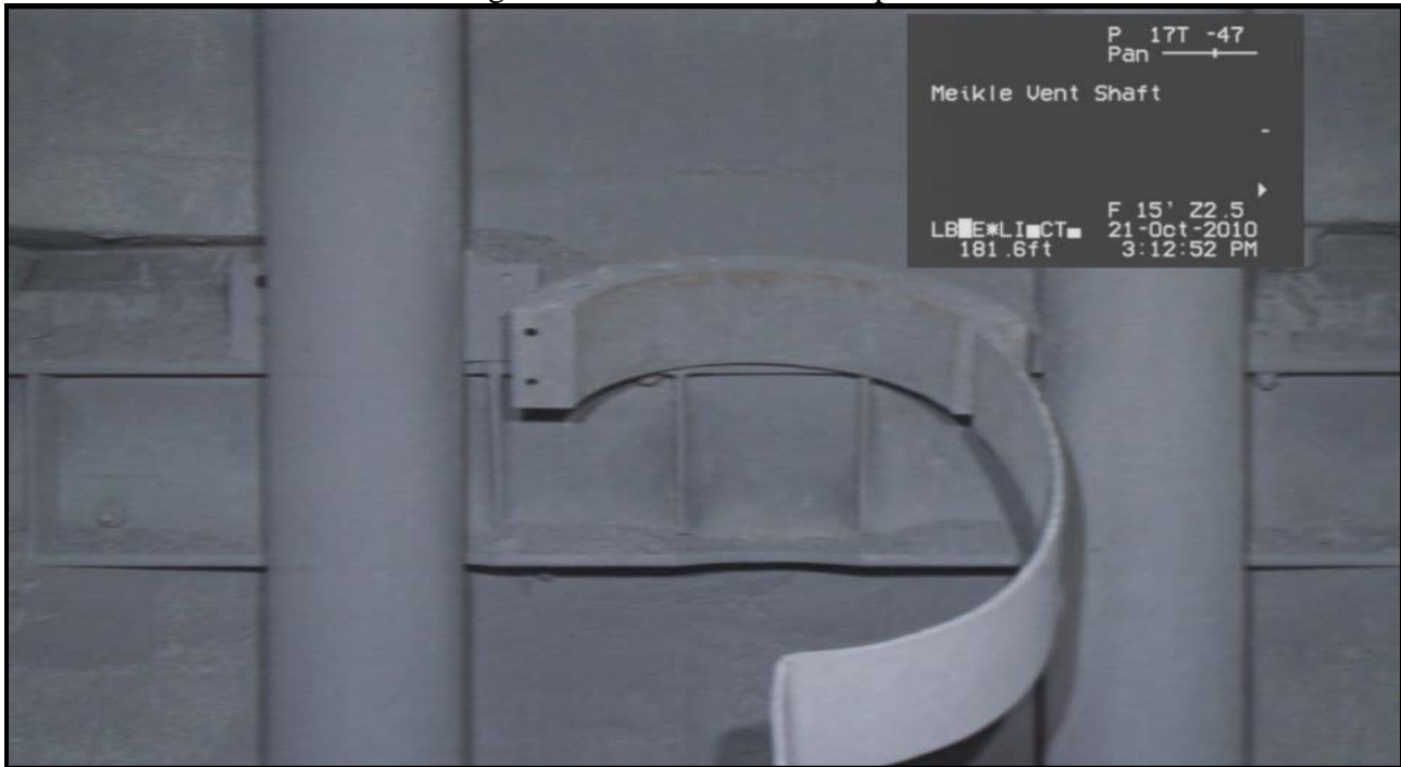
Photo 19 - Video Time 26:26 - Original bracket with one clamp bolt sheared.
