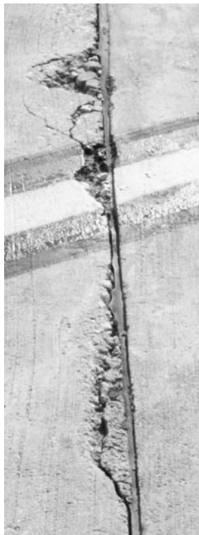
◀ Spalling along a joint.
