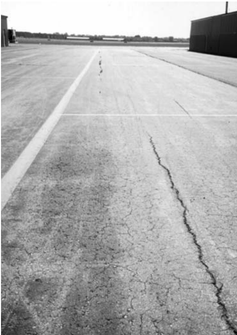
▶ Severe cracking and edge distress.
