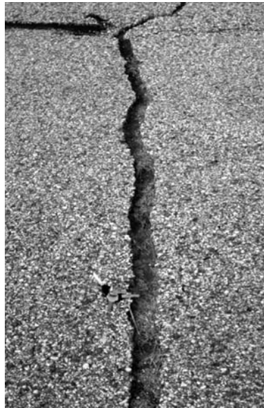
▲ Wide cracks with no sealant.
