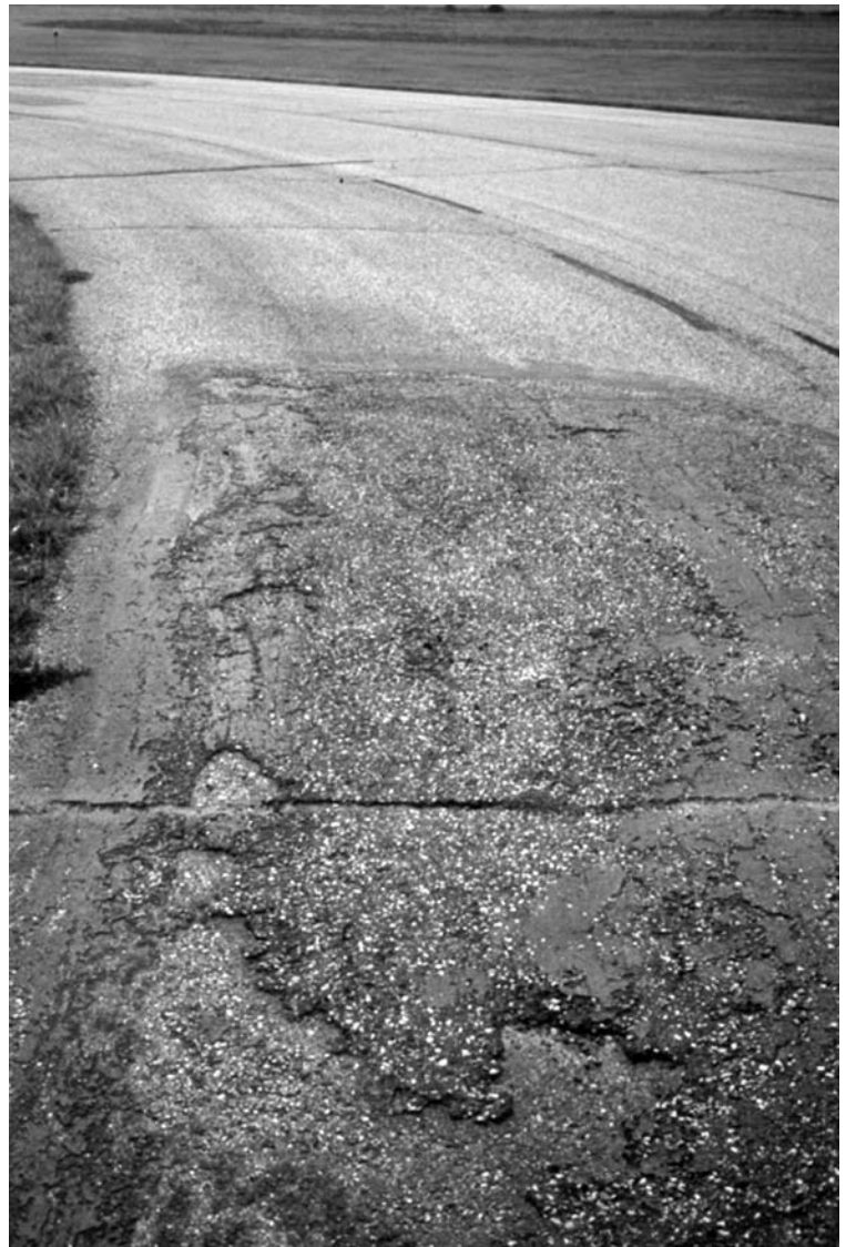
▶ Patched area in poor condition.
