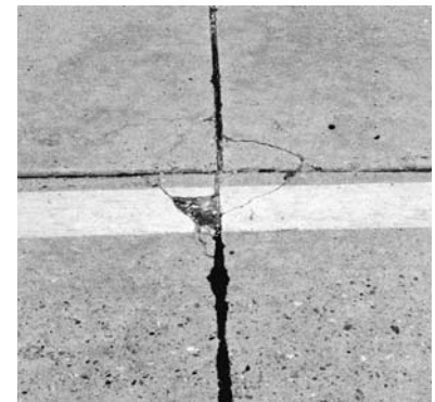
Corner cracking in all four slabs.
