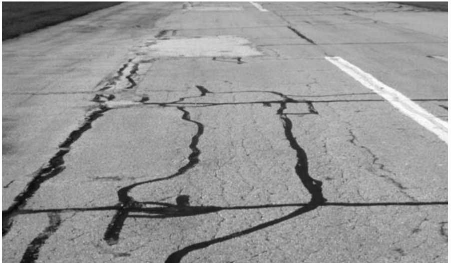
▲ Extensive alligator cracking. Poor patches.
