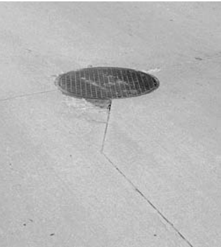
▲ Isolated spall at manhole.
