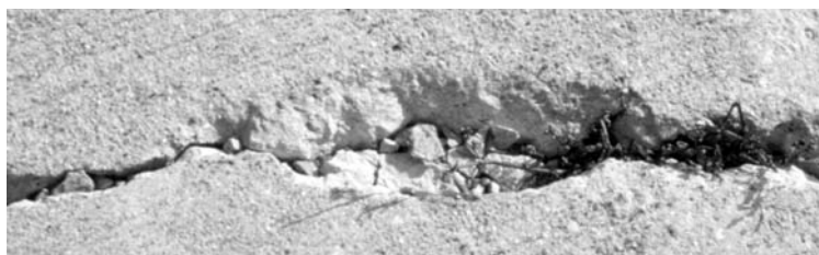
◀ Spalling along a joint.
