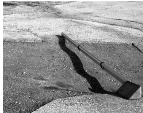
▲ Frost heave damage from spring break-up.
