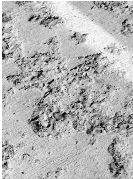
◀ Severe scaling. Some larger aggregate is loose.
