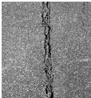
▲ Wide cracks with no sealant.
