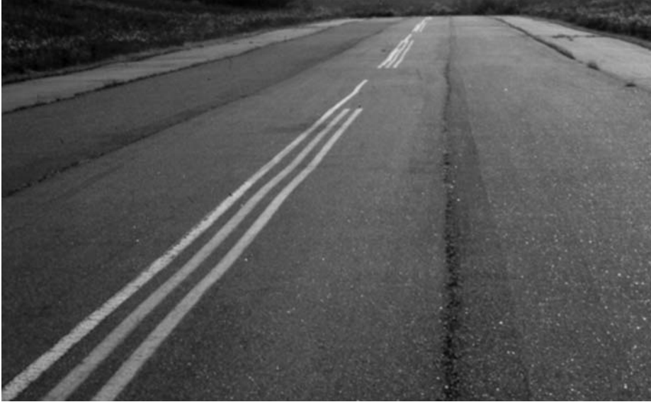
▲ Paving joints. Slight crack on joint near center. Open joint on right side.
