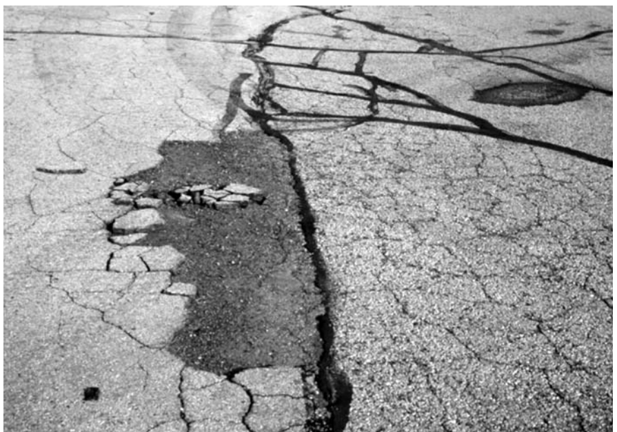
▶ Extensive failed pavement and debris.
