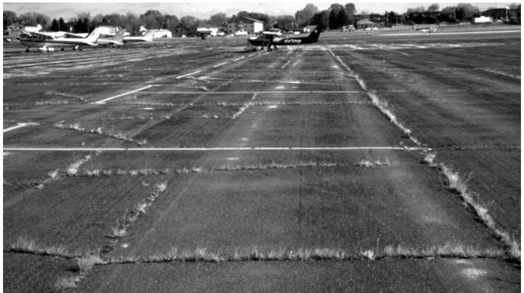
▶ Right angle cracking forms blocks.
