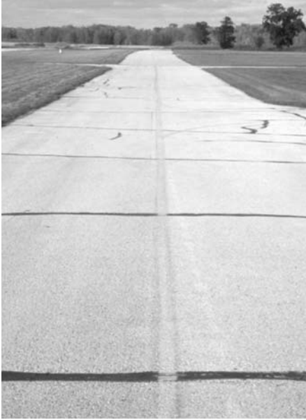
▲ Widely spaced, well-sealed cracks.
