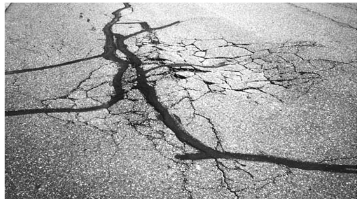
▲ Frost heave damage from spring break-up.
