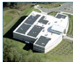
Photovoltaics sit on the "cool roof" of the Environmental Protection Agency's Research Triangle Park facility.
