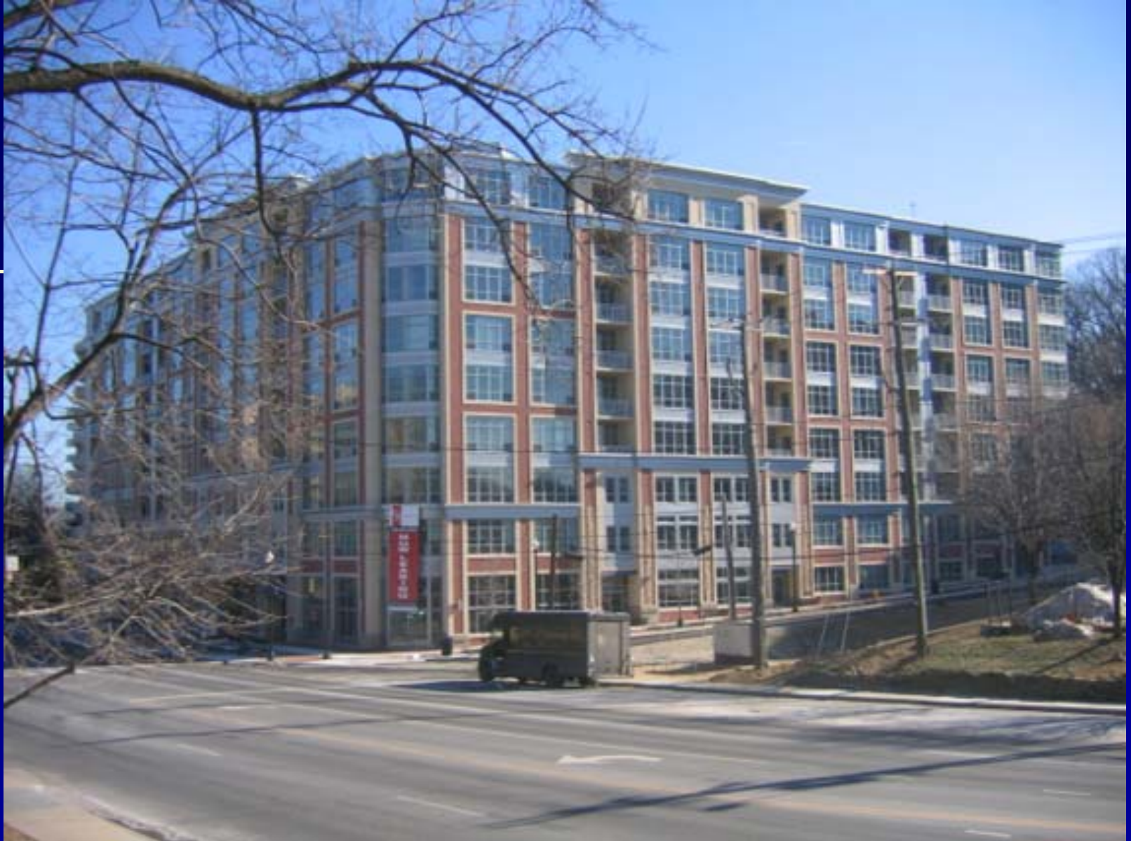
The just-completed project, winter 2010
