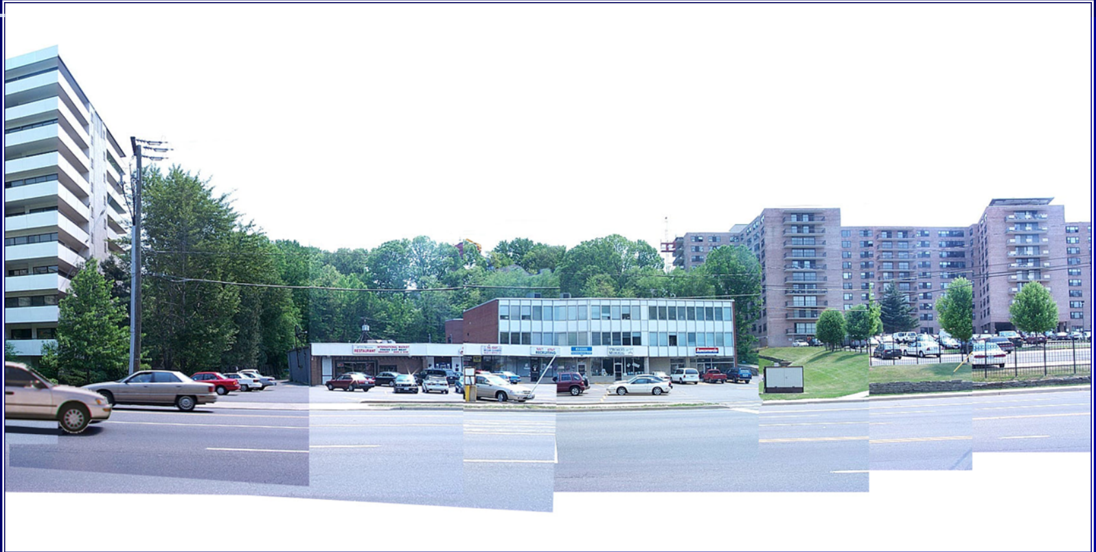
Small strip commercial building with surface parking lot, circa 2002
