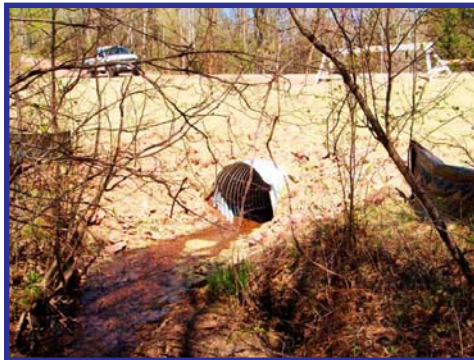
The Billy Creek fish passage project was completed in Ashland County, Wisconsin. The old road culvert was impassable (above). The new culvert (below) provides uninhibited fish passage.
