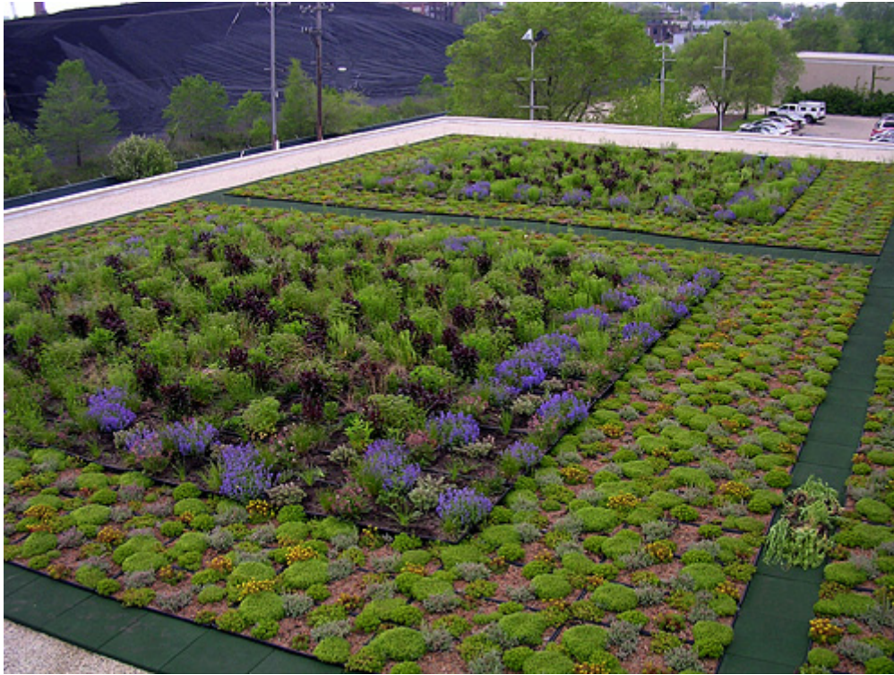
FIGURE 14: Example of modular drop-in-place system. 20
