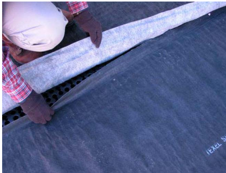
FIGURE 8: Filter fabric installed over plastic drainage layer. 14
