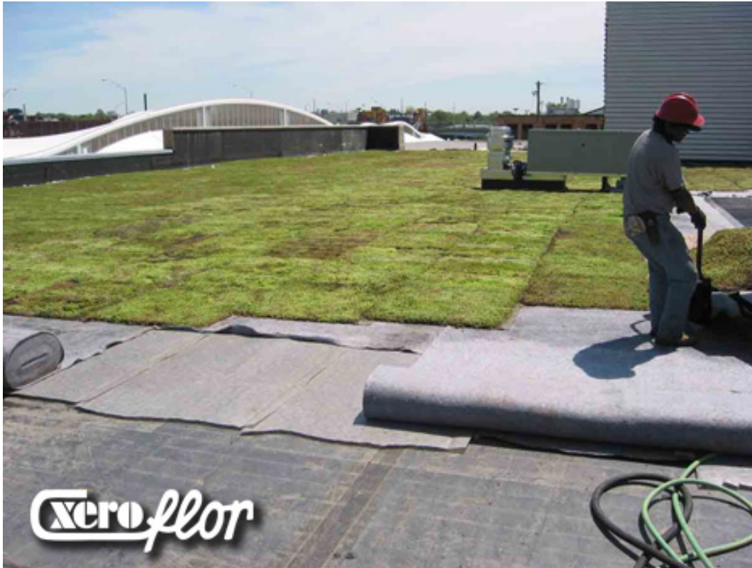
FIGURE 9: Example of pre-vegetated mat. 15
