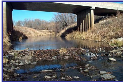
Fish Passage funding contibuted to modifications on Turkey Creek in Cass County, Iowa. The above weir has a 4:1 slope. The below photo is the reconstructed water control wier with a 15:1 slope which approximates natural stream gradients.
