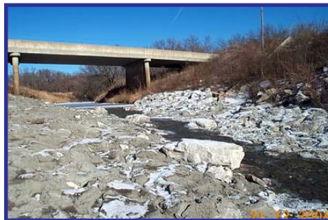
Fish Passage funding contibuted to modifications on Turkey Creek in Cass County, Iowa. The above weir has a 4:1 slope. The below photo is the reconstructed water control wier with a 15:1 slope which approximates natural stream gradients.
