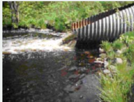
As part of fish passage projects, perched culverts (left), are replaced by boxed (right) or other similar culverts that allow the free movement of fish and other aquatic species.
