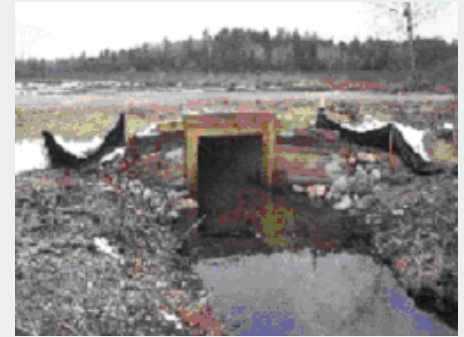
As part of fish passage projects, perched culverts (left), are replaced by boxed (right) or other similar culverts that allow the free movement of fish and other aquatic species.
