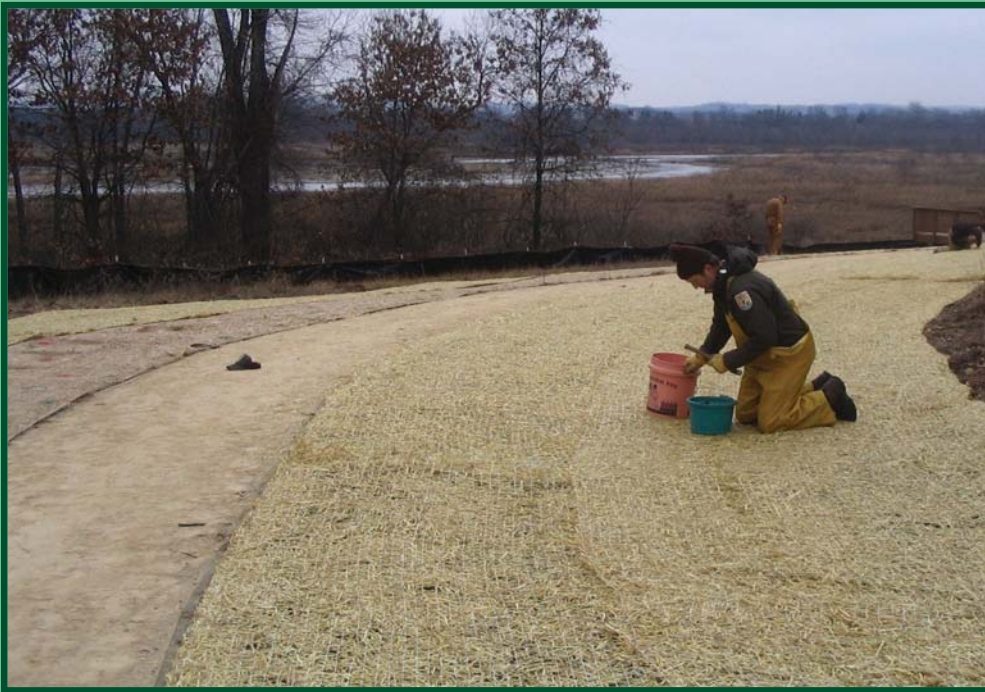
Above: Mark Steingraeber fights cabin fever by laying straw erosion mat to cover newly planted seeds. Photo by Calvin Gehri/USFWS.
