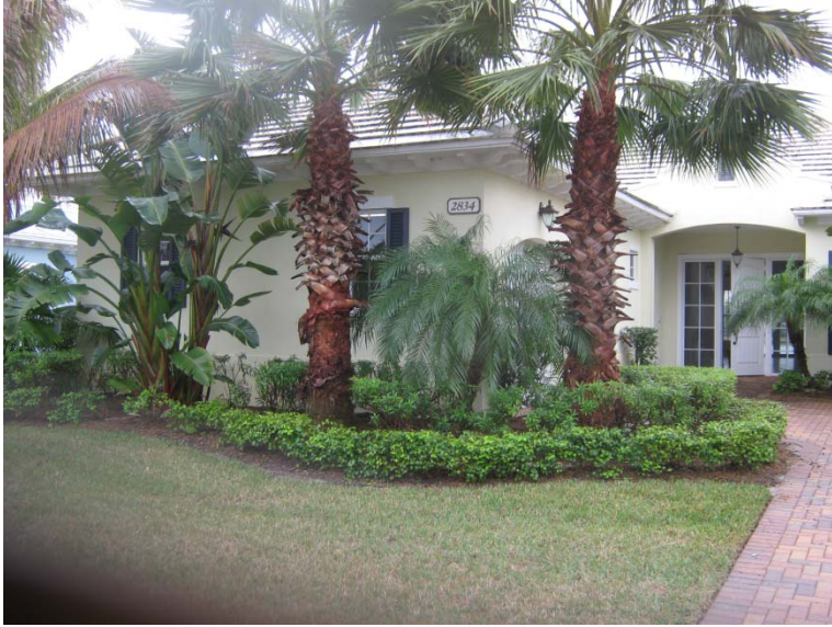
Exterior of the residence.
