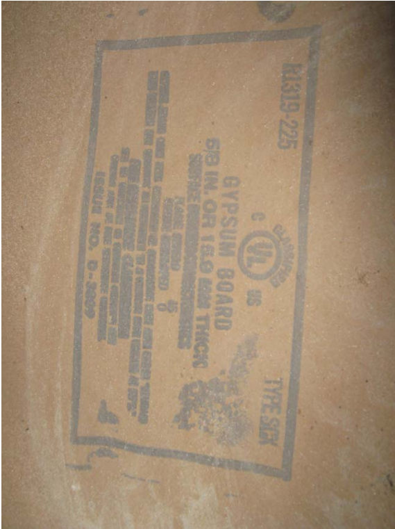
Wallboard label within the attic.
