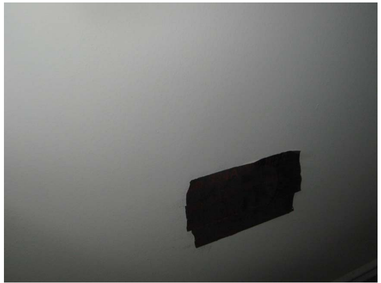
Core sample location behind the refrigerator.
