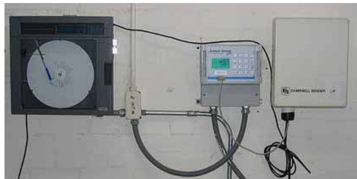
Figure 3.5. Circular Chart Recorder, Data Logger, and Internet Interface
