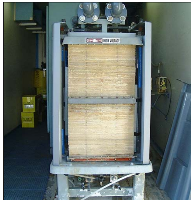
Figure 3-14. EDR stack.
