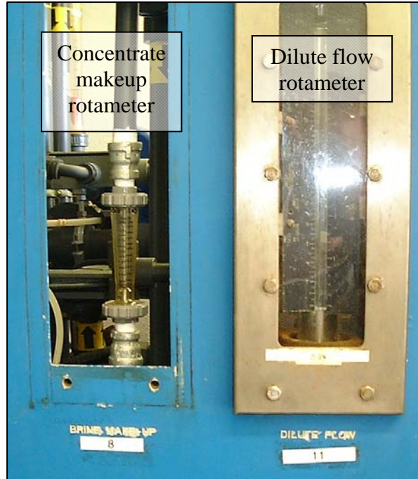
Figure 3-10. EDR rotameters.
