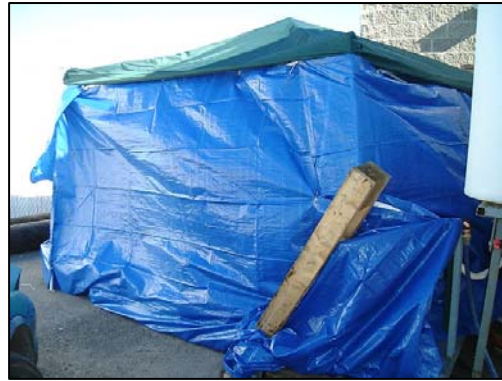
Figure 5-1. RO Pilot Tarp Enclosure.
